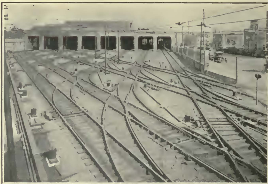
69th Street Terminal, Philadelphia, Pa.
