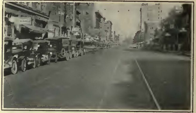
This Track Built with Dayton Mechanical Ties Has Stood Up Well Under Heavy Traffic for Seven Years
