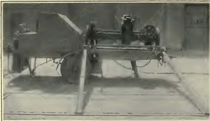
This Trail Truck Has Been Designed by the Eastern Massachusetts Street Railway to Carry All the Machinery Needed for Small Track Construction Jobs
