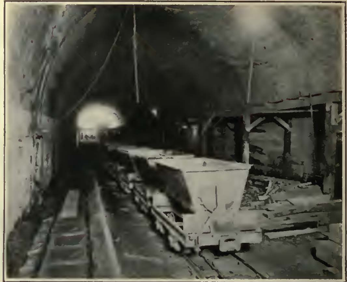
At Left—By Working 24 Hours a Day in Three Shifts the Railway Has Been Able to Dig the Subway at a Speed of About 30 Ft. a Day. At Right—Excavated Material Is Carried from the Bore to the Foot of the Hoist by a Light Railway
