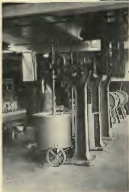
Portable Paint Mixer—An 80-Gallon Tank, One of Twelve Units in the Everett Shops, Is Shown on the Truck
