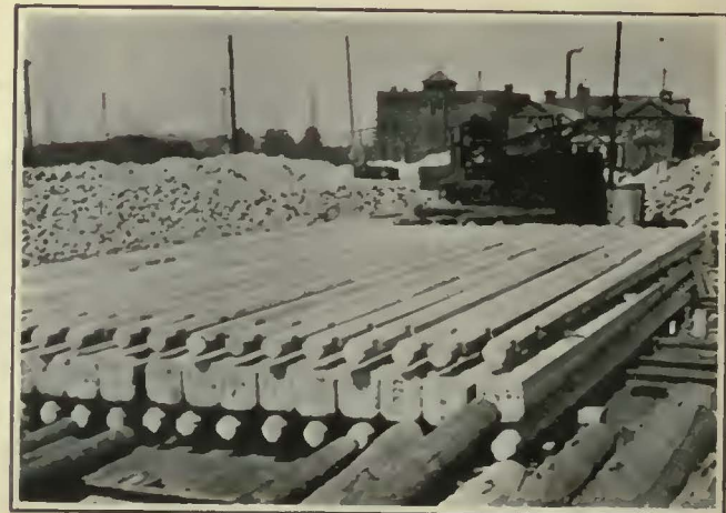
Method of Storing Concrete Poles in the Yard of the United Railways of St. Louis
