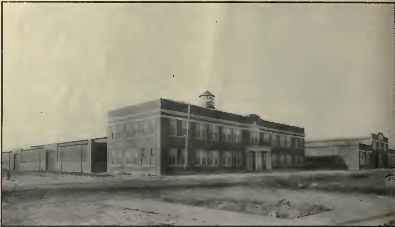
General view of new, complete terminal of The Detroit Motorbus Co., Dexter Blvd., and Penna. R. R. Architectural design, construction and equipment by The Austin Company. This Terminal is comprised of Administration Building, Body Shop and Garage.
