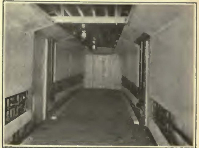
Interior of the Refrigerator Car. It Is Thoroughly Insulated Against Heat. A Thermostat Near the Center Is Set to Regulate the Temperature
