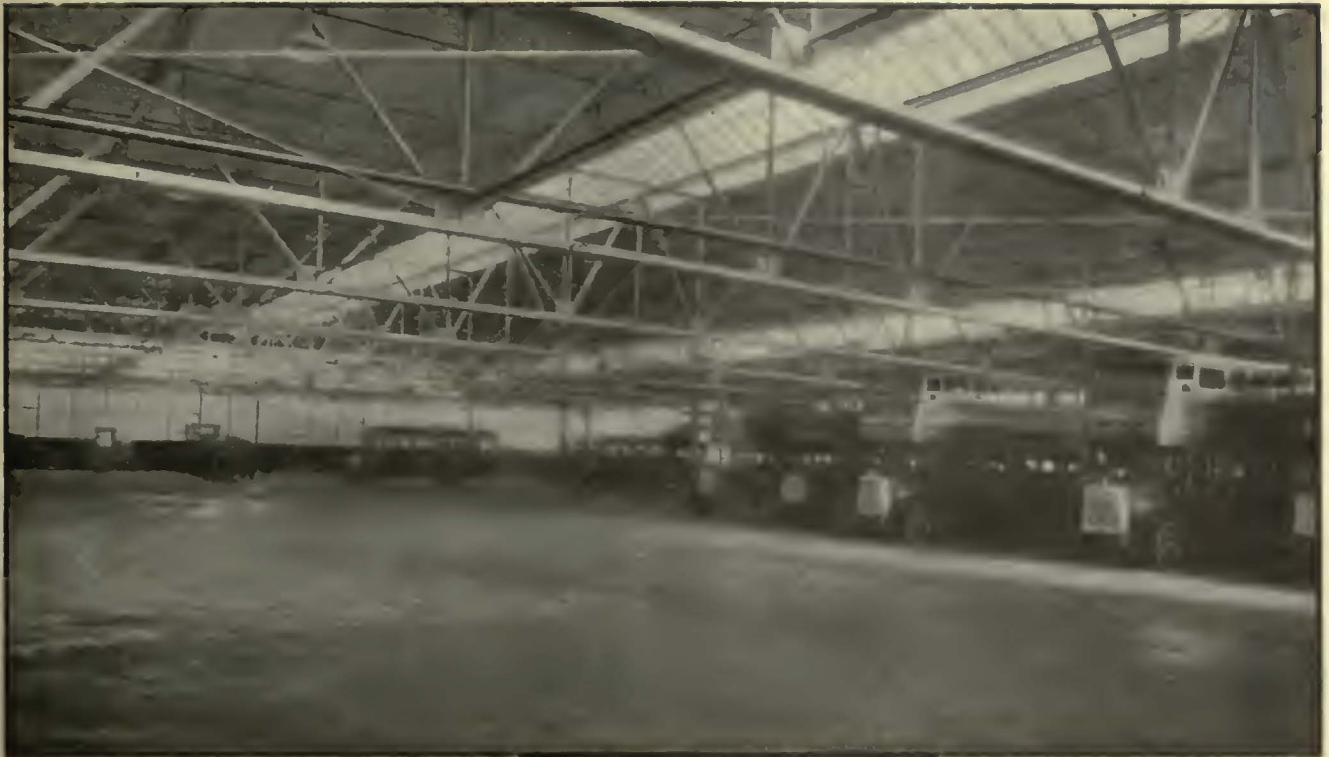
Interior of the well daylighted and ventilated garage at the Detroit Motorbus Terminal at Dexter Blvd., and Penna. R. R. Capacity, 100 double-deck buses. The building also contains an aisle for running repairs. Underground fuel storage has a 35 tank car capacity.
