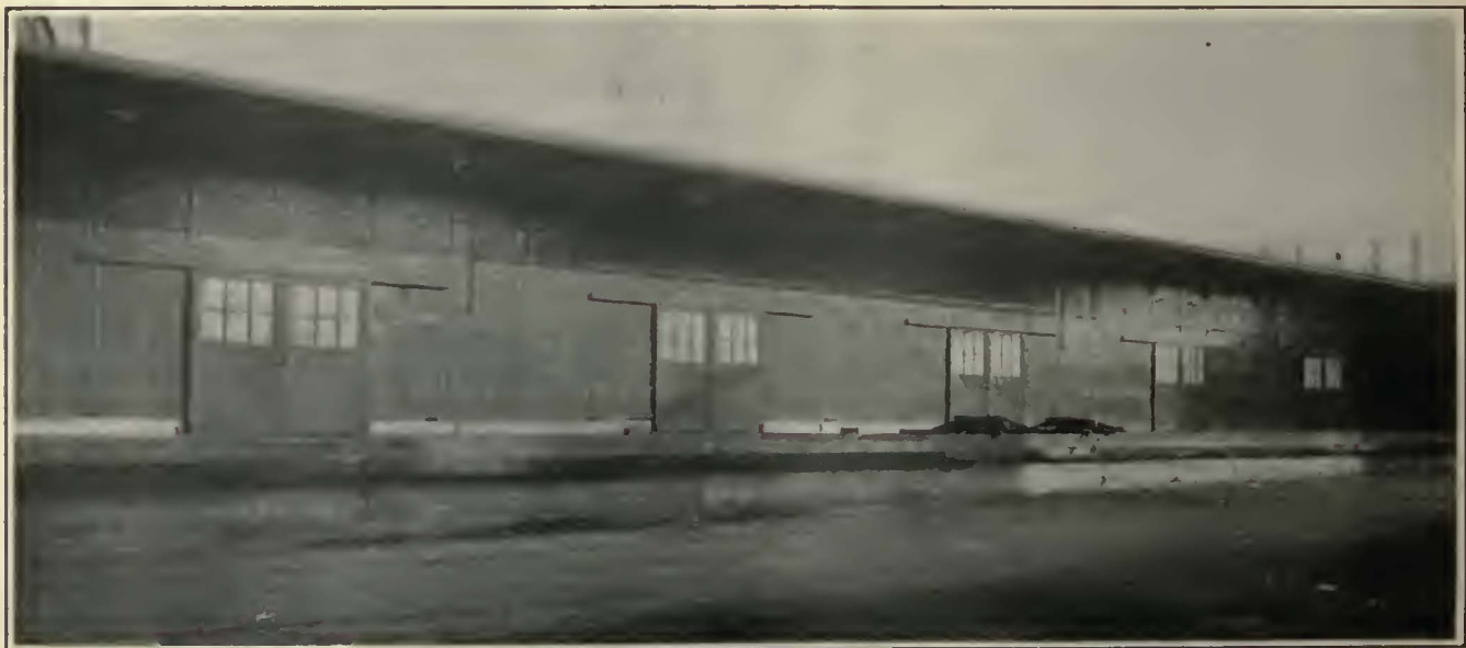
The Loading Platform Extends the Length of the Fireproof Sheet-Metal Warehouse and Is Served by a Double-Team Track
