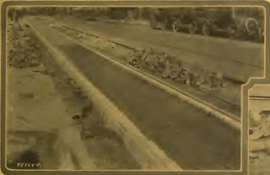
At left—Pennsylvania Avenue, Indianapolis, Ind. Installing Carey Rail Filler.
