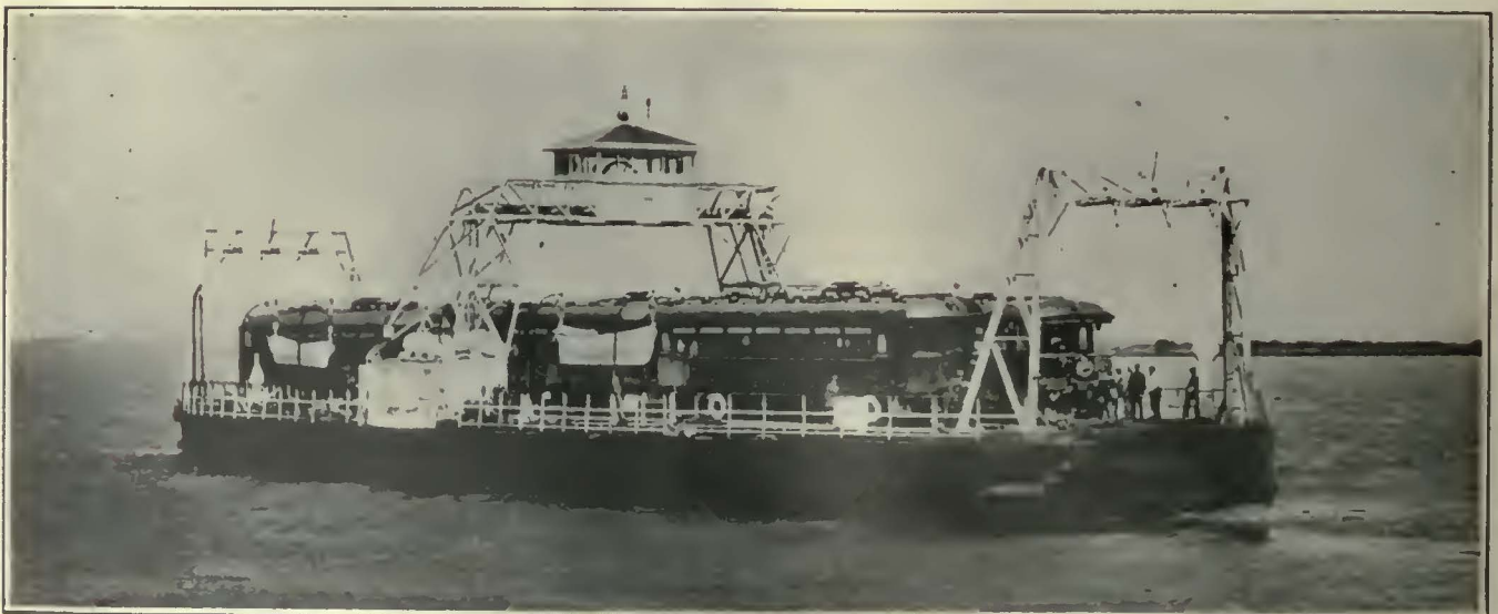
All Trains of the San Francisco-Sacramento Railroad Cross Suisun Bay on this Gasoline-Driven Car Float
