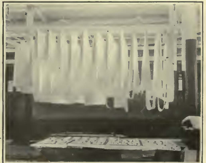
The Shade Cloth on Which Signs Are Printed is Treated in Advance with Fish Oil
