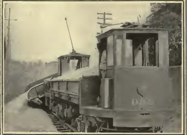
"Differential Two-Cor Train. Trailer dumping load clear of trench."
