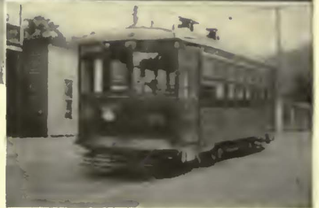
Hyatt bearings in the journal boxes of this car are effecting a 20% power saving for the Citizens Traction Company, Oil City, Pa.
