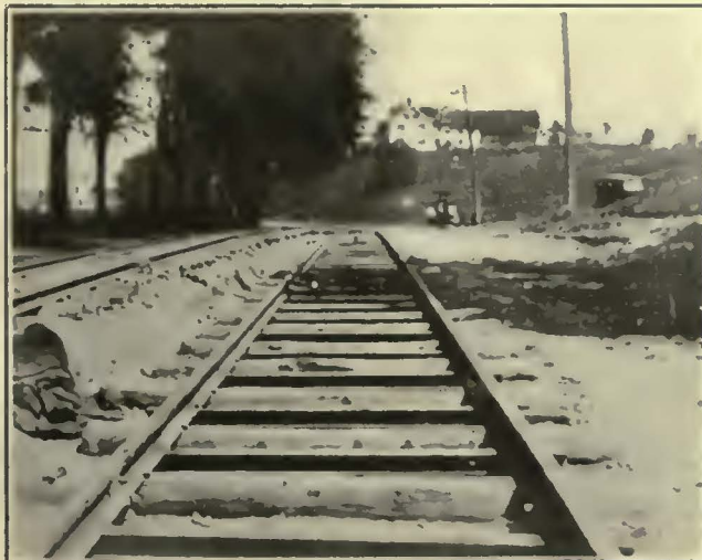
Joints Welded and Track Ready for Concrete
