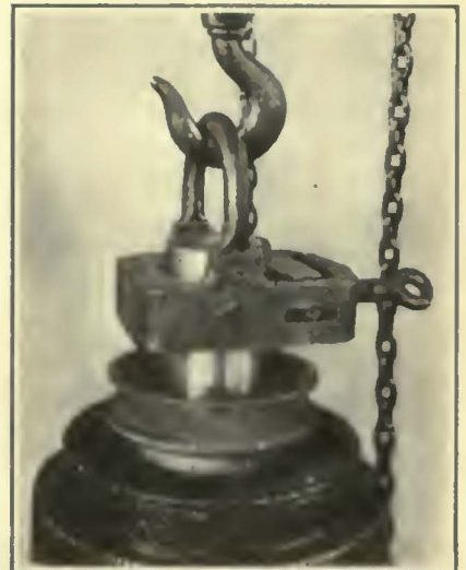
Clamp Applied to Armature Shaft to Support It in Vertical Position
