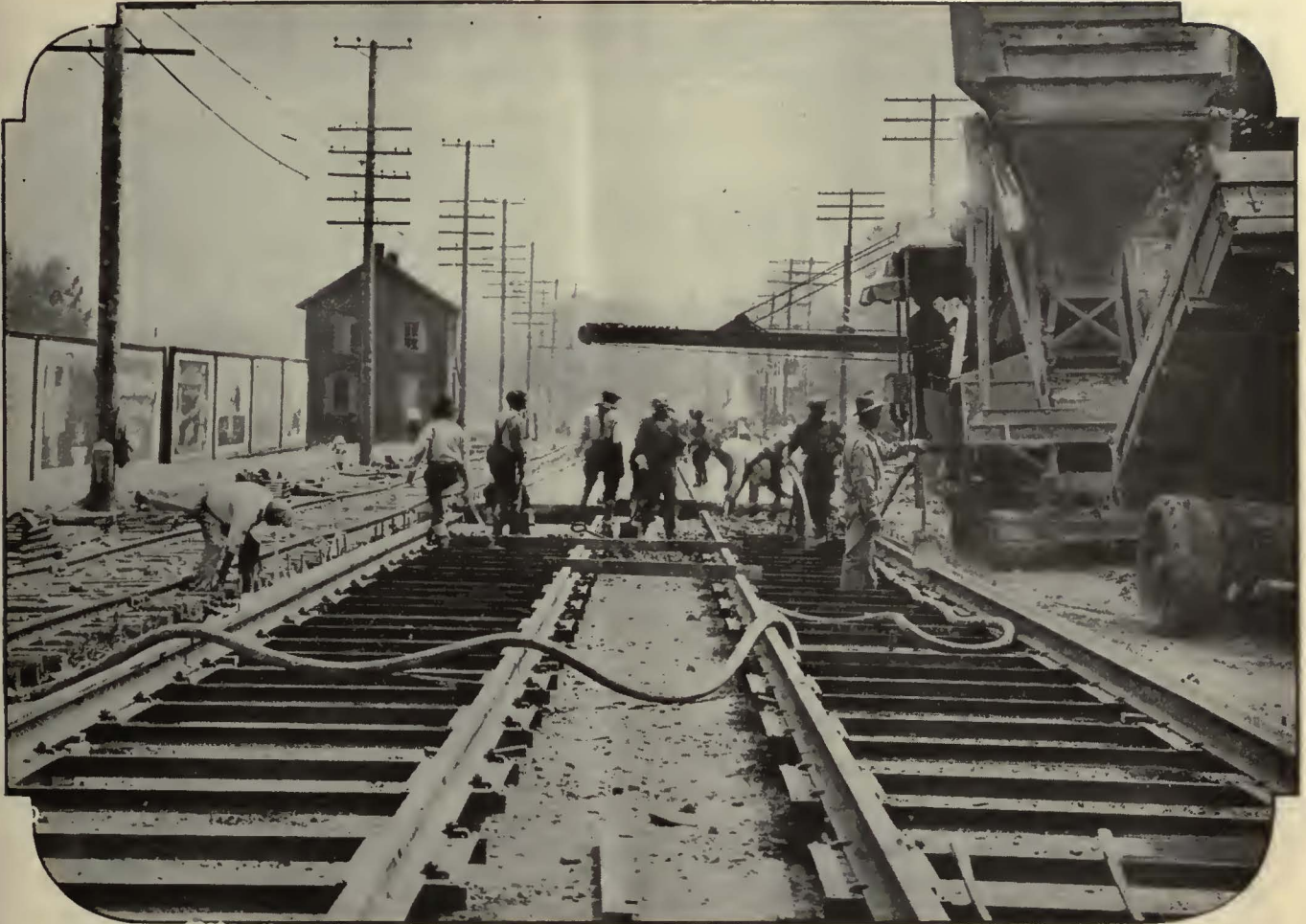
Double Track Reconstruction, Lancaster Ave., Reading, Pa.
