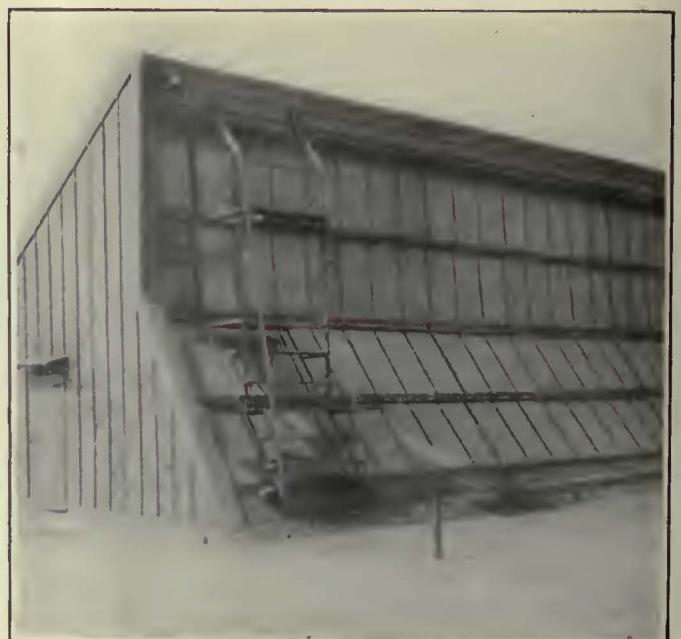
Skylight Scaffold Used at Everett Shops of Boston Elevated Railway
