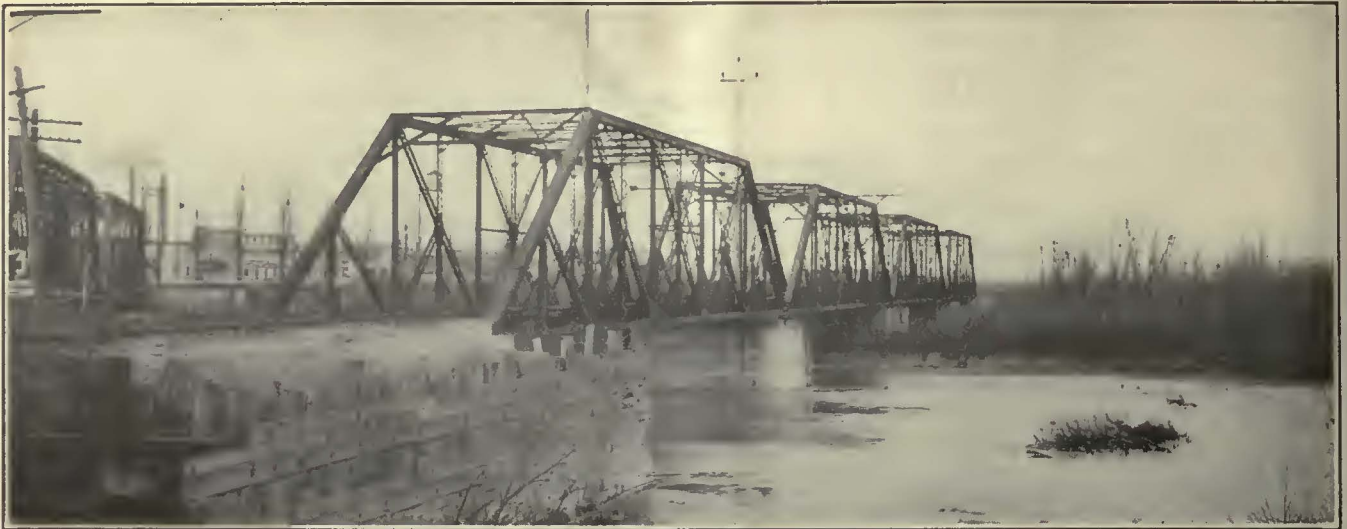
The Buffalo & Erie Railway Has Built Up a Profitable Business by Giving High-Speed Service Between Buffalo & Erie with Modern Light-Weight One-Man Cars. This View Shows a Bridge Over Cattaraugus Creek at Irving, N. Y.
