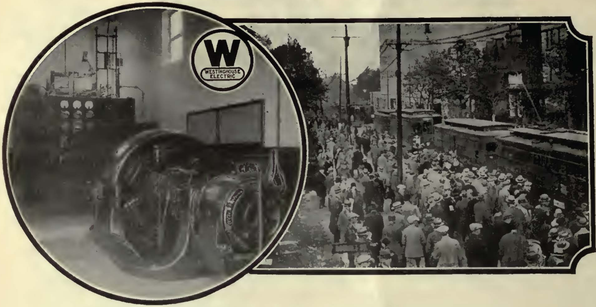
A Westinghouse automatic substation recently installed by the Connecticut Company at Branford, Connecticut.
