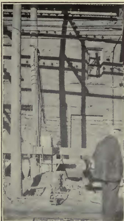
At Left, Shoring Up Poles After Old Butts Had Been Cut Off. In Center, Lowering New Concrete Base Into Position. At Right, Malleable Iron Castings Were Used to Hold Poles in Place
