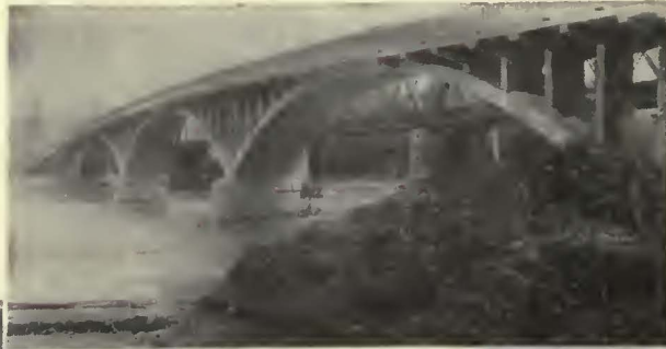
Humboldt County Van Duzen River Bridge View looking North.
