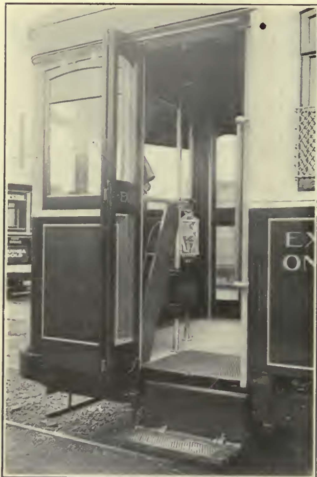
Treadle and Step of Automatic Rear Exit on Toronto One-Man Cars
