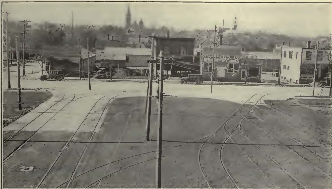
Reconstructed Entrance to Carhouse of Wisconsin Power & Light Company's Property at Sheboygan, Wis. Sidewalk, Curb and Gutter Have Been Eliminated to Provide Easy Access to Yards for the Company's Buses
