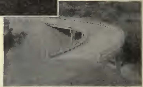
Bridge over North Fork Pacheco Creek. Located in Santa Clara County
