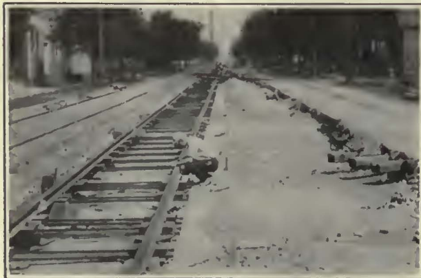
Views Showing Reconstruction Work at Sheboygan by the Wisconsin Power & Light Company. At Left Is the Temporary Track Used During Reconstruction. At Right Is a Stretch of Finished Track Alongside of a Short Section Ready for Concreting
