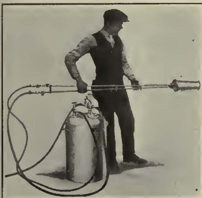
New Atomizing Type of Oil Burner and Preheater
