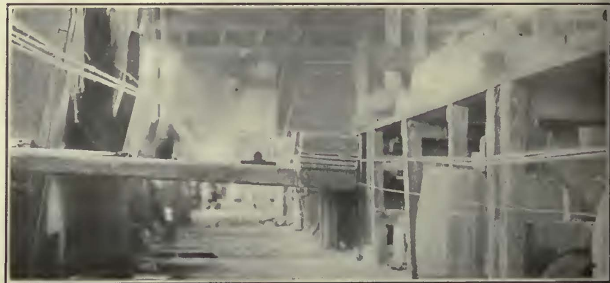
Armature Winding Wires Pass Between Fiber Plates Bolted to the End of a Wooden Arm
