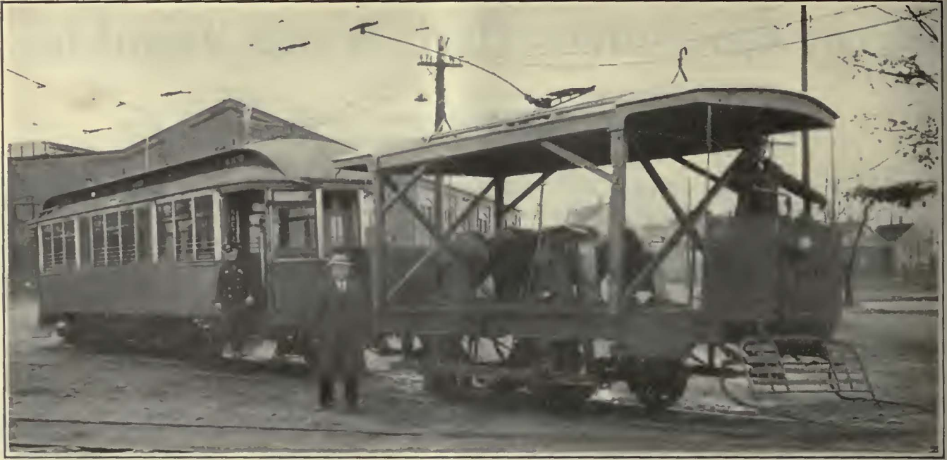
A Special Motor Car with Motors Mounted Above the Floor Hauls a High Platform Trailer
