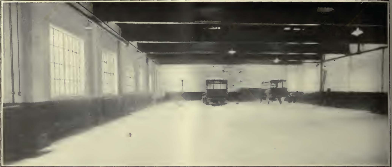
Substitution of Steel Beams for Wood Posts Has Permitted the Dubuque Electric Company to Transform an Old Carhouse Into a Roomy Garage
