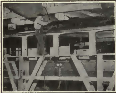
Applying a Coat of Paint to the Roof
