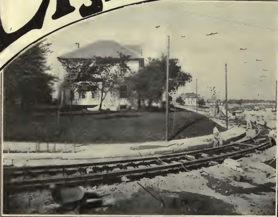
Photo when Dayton Ties were being installed in 1917.
