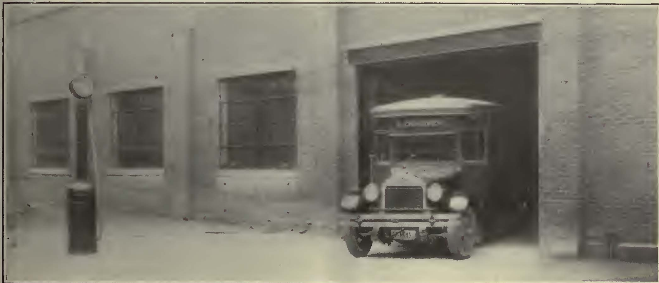
Entrance to the Garage Is Through an Adjoining Vacant Lot Which Has Been Graded and Paved with Concrete
