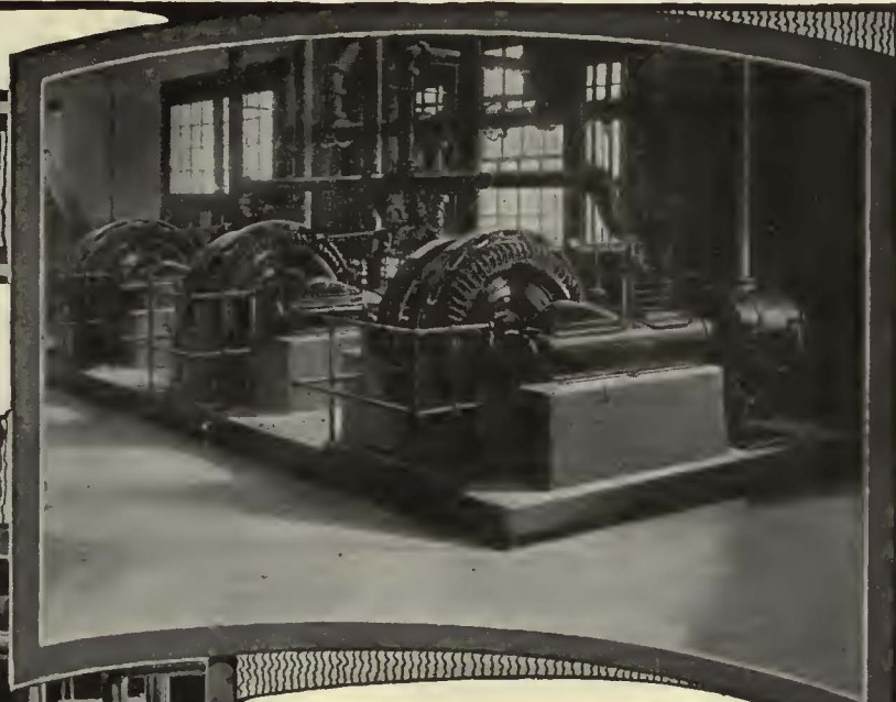
Right—Battery of Ingersoll-Rand single-stage direct connected electrically-driven air compressors for low pressure air.
