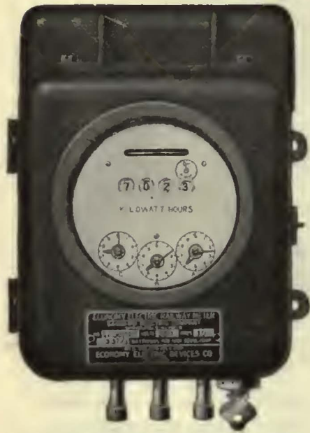
Economy Meter with Power Saving and Car Inspection Dials
