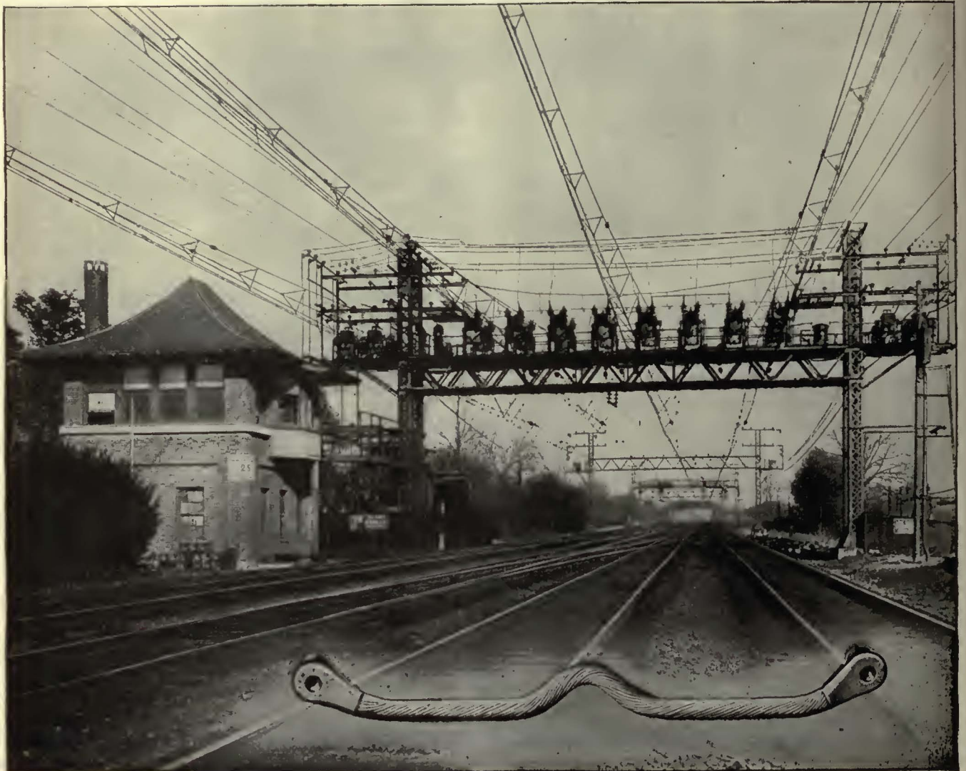
View of main line New York, New Haven and Hartford Railroad. Insert is our type CPOF Bond a concealed type of bond which is used on all main line tracks.
