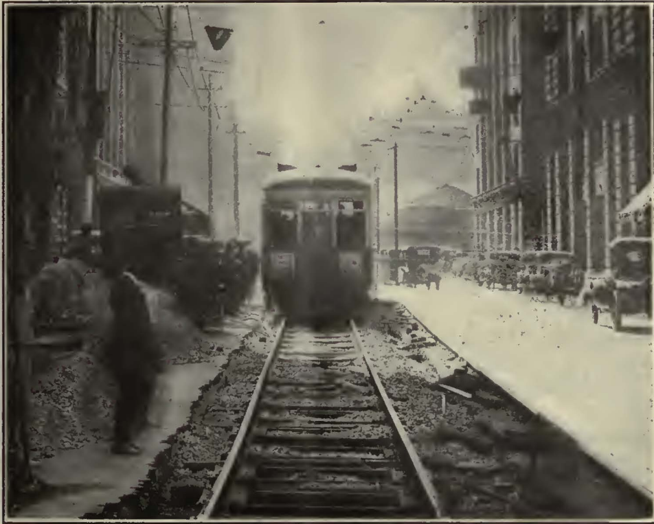
Twin Ties Being Installed Under Traffic in Kansas City
