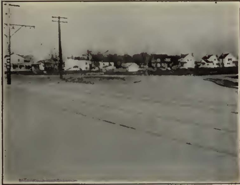
Wisconsin Avenue Circle, Washington, D. C., where concrete was laid by the District of Columbia and, with the aid of Cal, was opened to traffic in six days.
