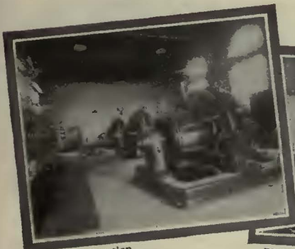
Rosindale Substation Boston Elevated Railroad One 2,000 and two 1,500 kw. Synchronous Converters
