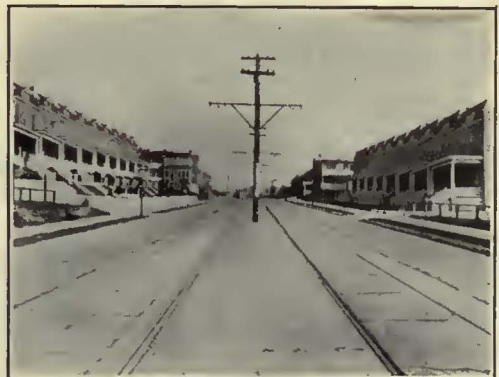
Upshur Street, Washington, D. C., showing Washington Railway & Electric Company's line where, with the use of Cal, concrete was laid while cars were in constant operation.
