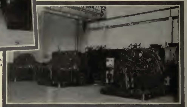
Mt. Vernon Substation Philadelphia Rapid Transit Co. Three 2,000 kw. Westinghouse Synchronous Converters
