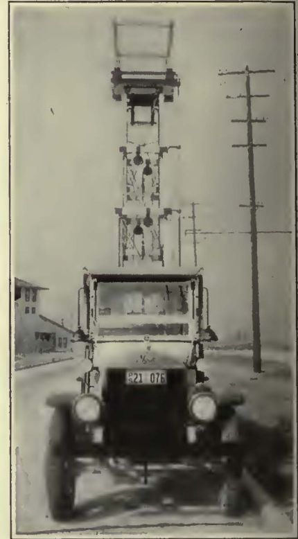
The Tower in Its Raised Position Provides for Work on the Highest Part of the Line and the Workmen Are Protected by Rallags
