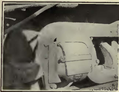
Strap Clamp Used by Union Street Railway to Hold Journal Box Covers in Place
