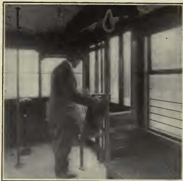
At Left—The Interior Finish Is of Mahogany. Ten Reversible Seats Are of Wood Slat Construction. At Right—A Book Type Folding Seat Provides Additional Seating on the Rear Platform
