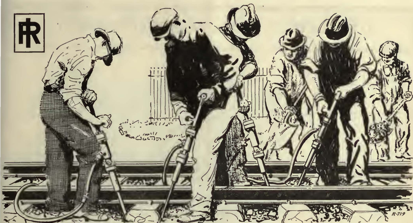
Four-tool Pneumatic Tamping Gang
