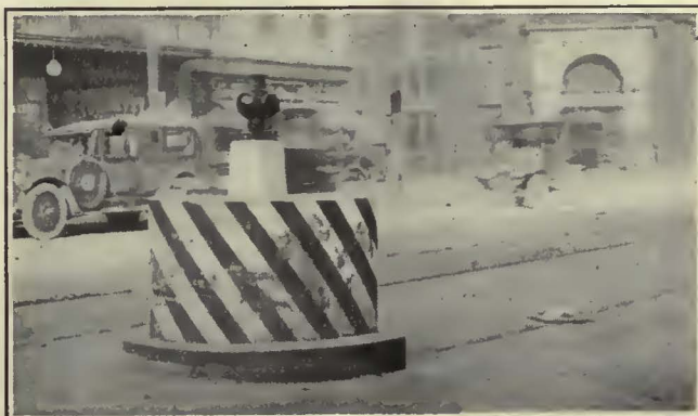
Reinforced Concrete Guard at End of Safety Zone—Cast-Iron Buttons and White Lines on Pavement Mark Limits
