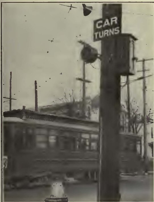
Signals in Connection with Floodlighted Signs Warn Motorists When Cars Are to Take a Turn. At Left, Pole Mounting for Sign. At Right, Pipe Bracket Mounting
