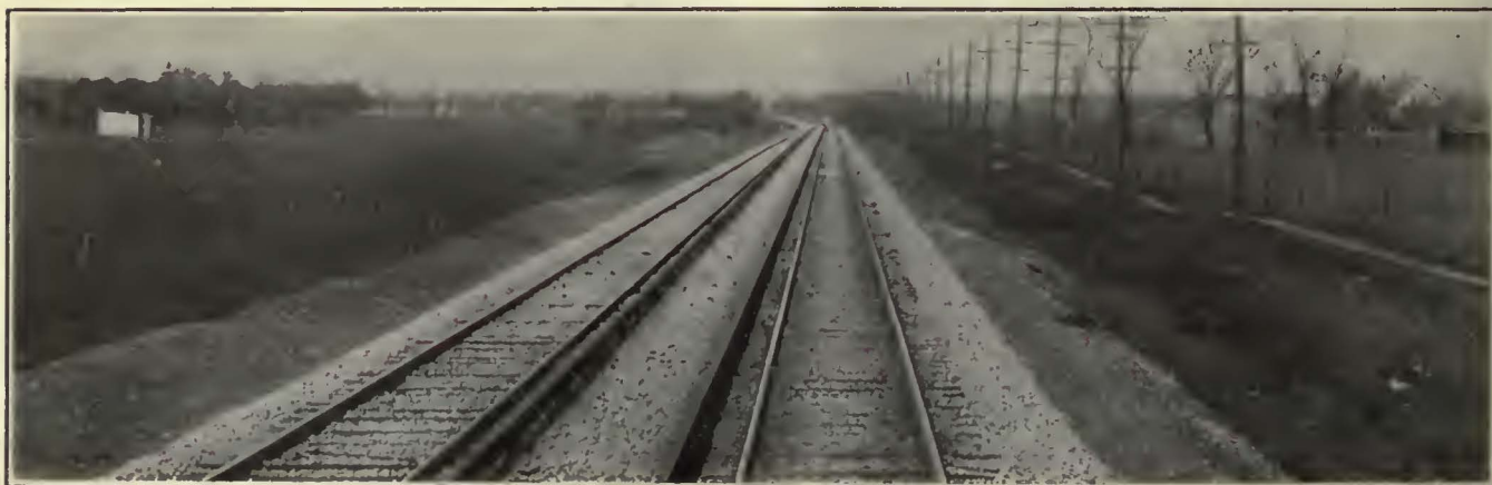
Well-Maintained Rock-Ballasted Track Permits High-Speed Operation
