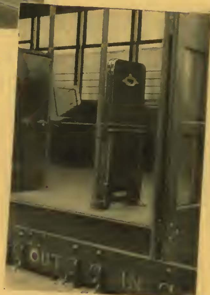
Separates incoming and outgoing passengers at service doors.
