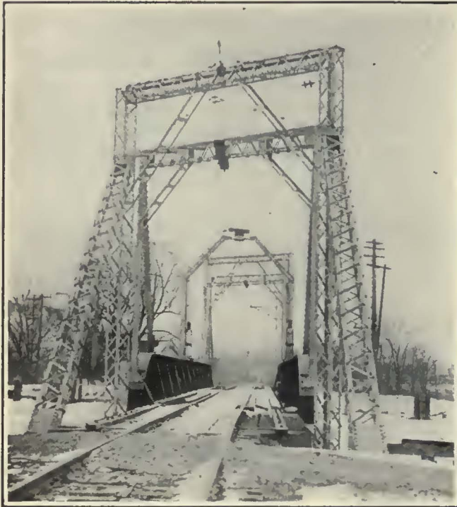
Overhead Structure at Welland Canal Swing Bridge
