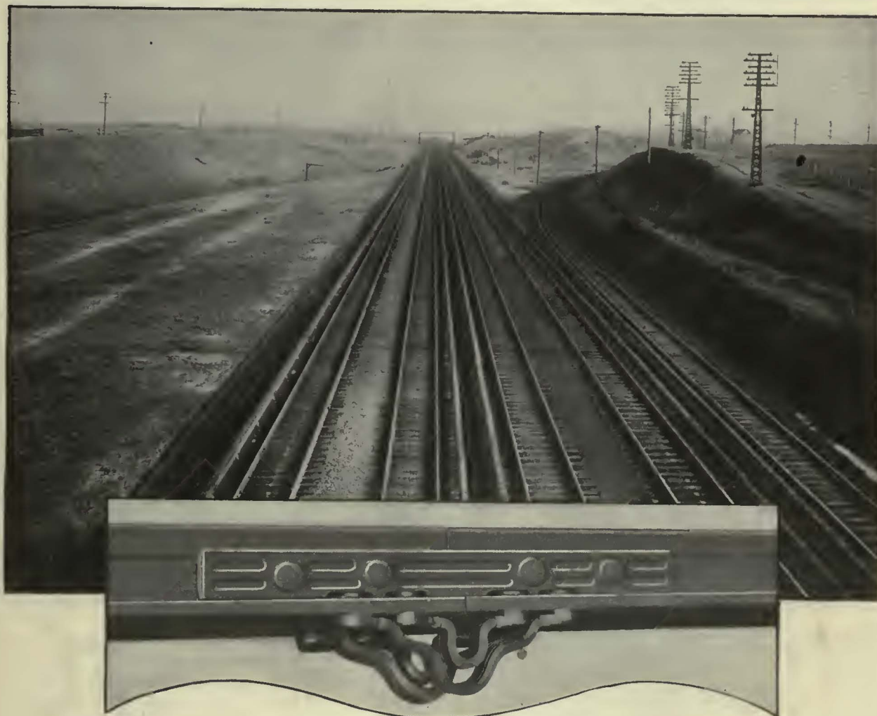
150 lb. Third Rail Joint bonded with 4—450,000 c. m. U. S. B. Bonds.
