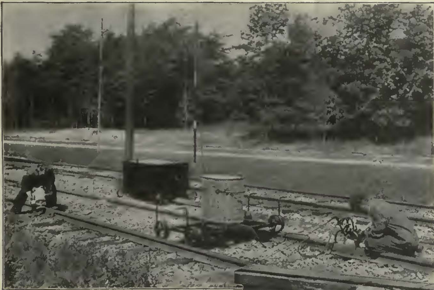
The Type SR Bonding Outfit installing Brazed Bonds on the head of rail.
