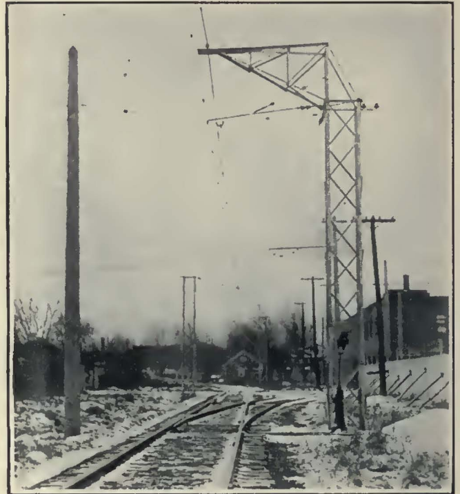
Standard Tangent and Armless Towers on Curve
