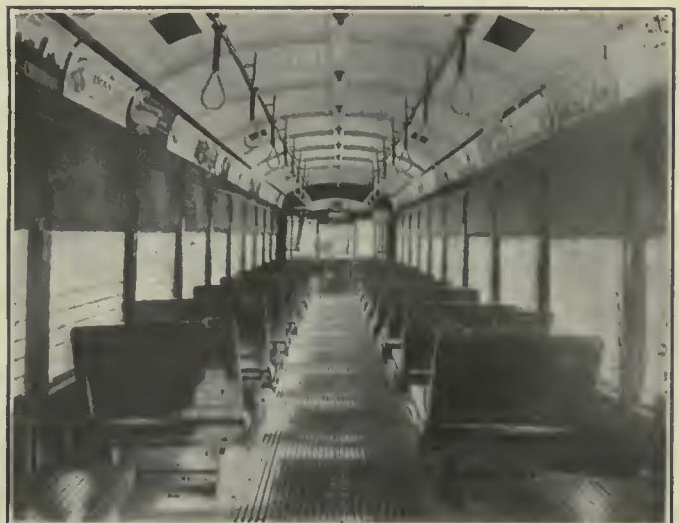
Interior Views of a Two-Man Car Changed Over for One-Man Operation. Dallas Plans to Change Over 50 of These Cars
