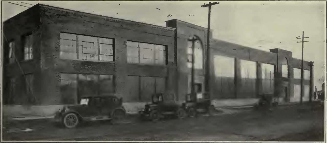
Combination Shop and Carhouse of the Aurora, Elgin & Fox River Electric Company Has a Steel Skeleton on Concrete Foundations with Brick Walls and a Wood Plank Roof
