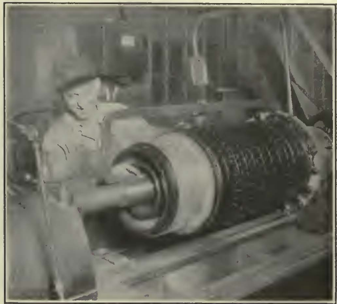
Measuring the Distance Between Wiper Faces of an Armature
