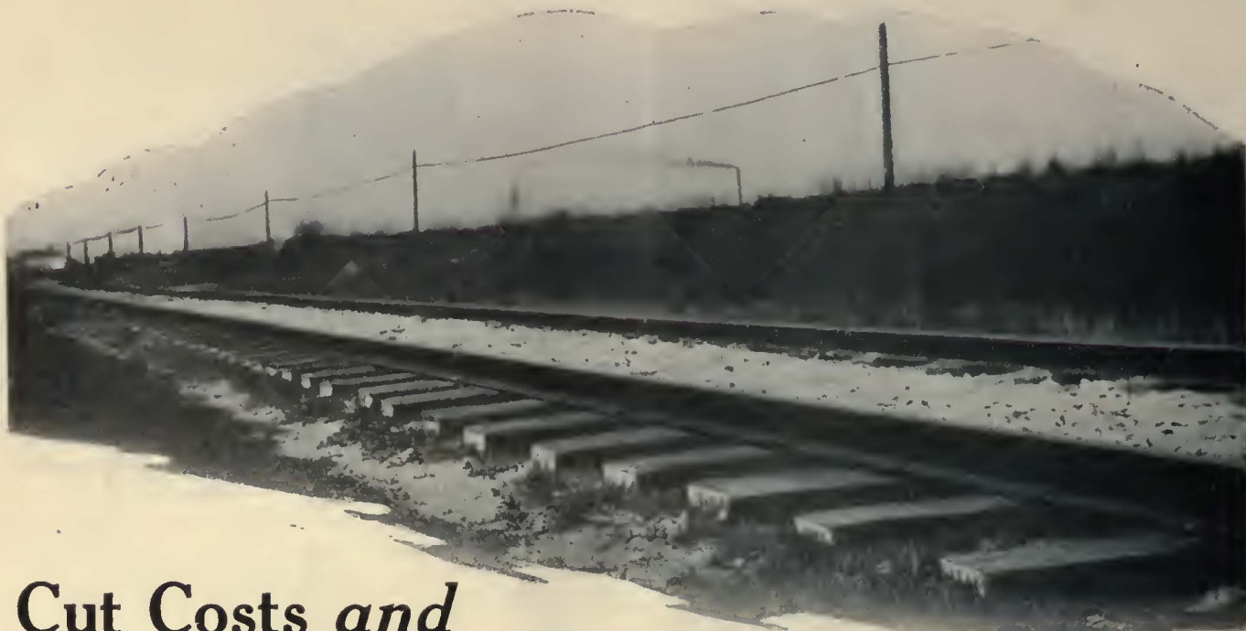
Port Arthur Traction Co. International Creosoted Pine Ties installed in 1909 in street car service in the city of Port Arthur, Texas.
