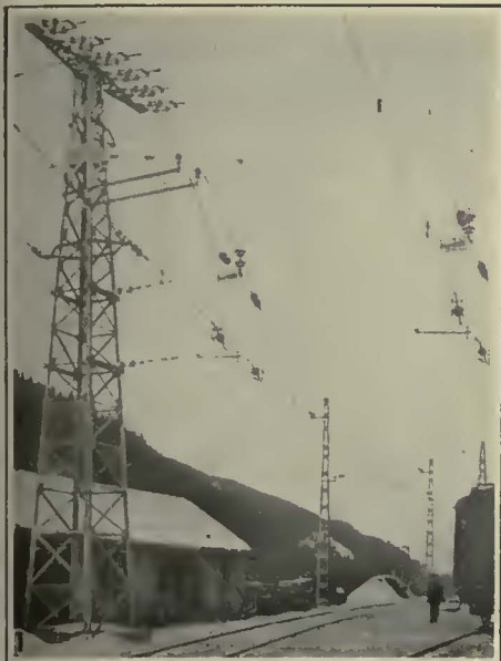
No. 1. A Typical Anchor Tower In a Switch Yard on the Arlberg Line. On This Section the Overhead Line Uses Suspension Insulators
