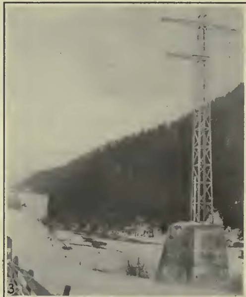
No. 3. The Transmission Towers Are Mounted on High Concrete Bases, at Points Where the Snowfall is Likely to Be Heavy
