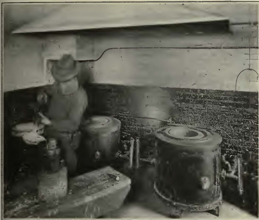
Thermostatic Control Provides Even Heating Temperatures for Atlanta Company's Gas Furnaces
