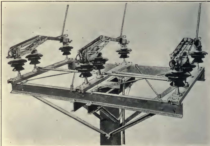
Pantograph Switch on Single Wood Pole Galvanized Steel Mountings
