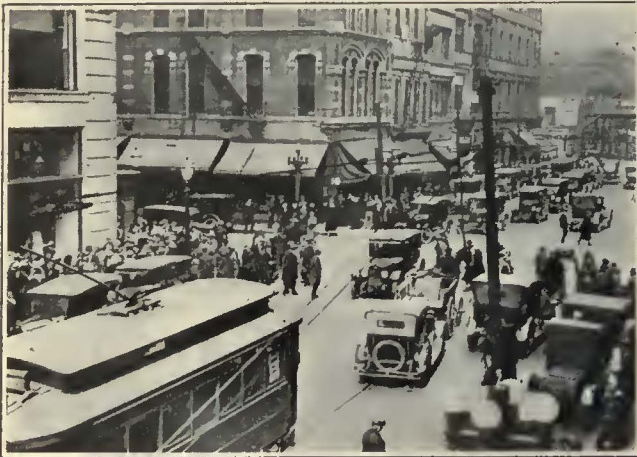
Traffic at Most Congested Crossings Is Now Controlled by Light Signals
