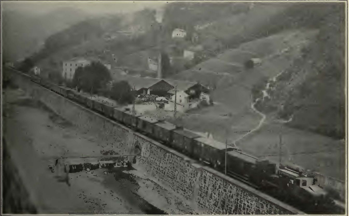
The Lower Giovi Line Handles Heavy Freight. The 400-Ton Train Shown Is Ascending a 3.5 per Cent Grade at 31 M.p.H.
