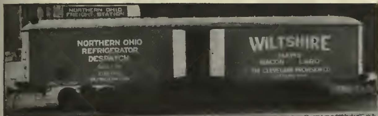
This is the first Phoenix Electric Refrigerator Car, converted from a standard freight car by The Northern Ohio Traction Co. It carries over 1,000,000 lbs. of perishable products in a year.
