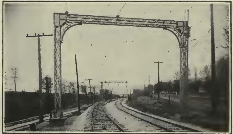
On curves of small radius, the overhead construction is carried by displaced catenary without pull-offs. In this particular instance, on a 7 deg. curve, the catenary is displaced 106 in.
