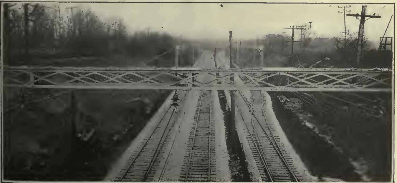
Where the New Skokie Valley Line Parallels the Old Libertyville Branch Line. The Overhead Bridges Span Four Tracks and in Some Cases Have a Length of 99 Ft.
