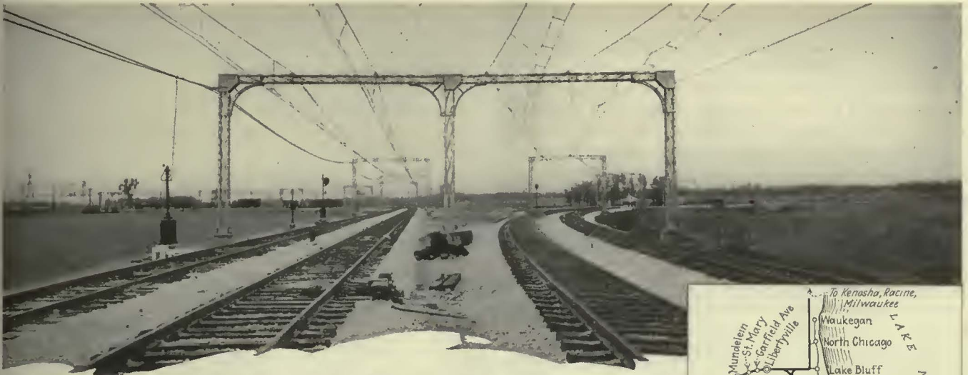
Skokie Valley Line of the Chicago, North Shore & Milwaukee Railroad Joins and Crosses the Libertyville Branch at a Wye at South Upton Junction
