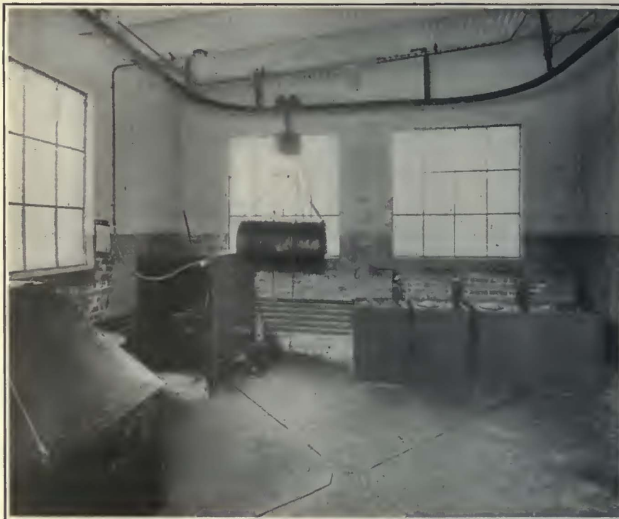
Construction of This Commodious and Well-Equipped Oil House by the Eastern Massachusetts Street Railway Has Gently Facilitated the Handling of Lubricants
