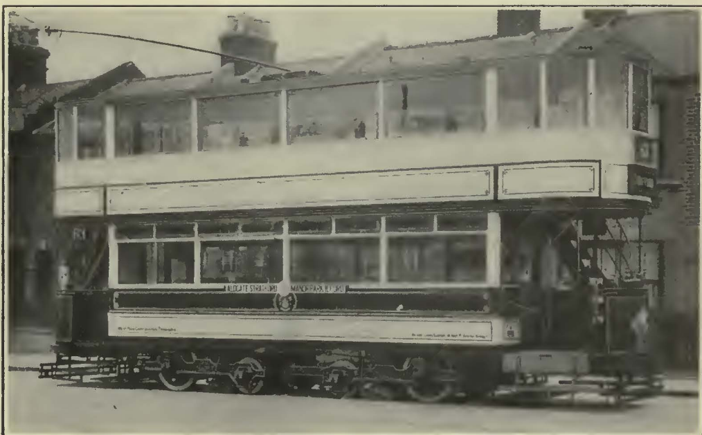
New Car of the West Ham Corporation Tramways Is One of a Comparatively Small Number of Double-Deck Vehicles Included in Recent British Orders. At the Left Is the End View of This Car, Showing Collision Bumper That Is Backed Up by Strong Spiral Springs
