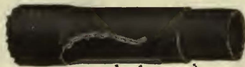
THE "WIRE LOCK" / / THE CHAMFERED JOINT
