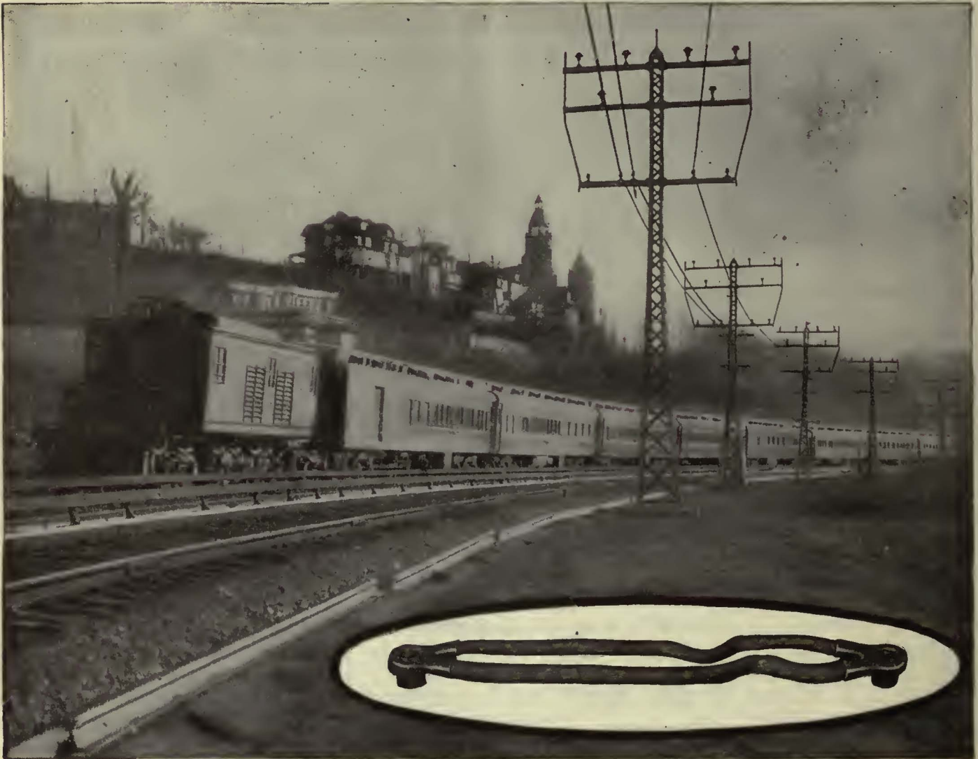
View of 20th Century rounding bend at Marblehead. The New York Central is always among the leaders in modern equipment. Insert shows our type CPO1 Bond used on all main line tracks
