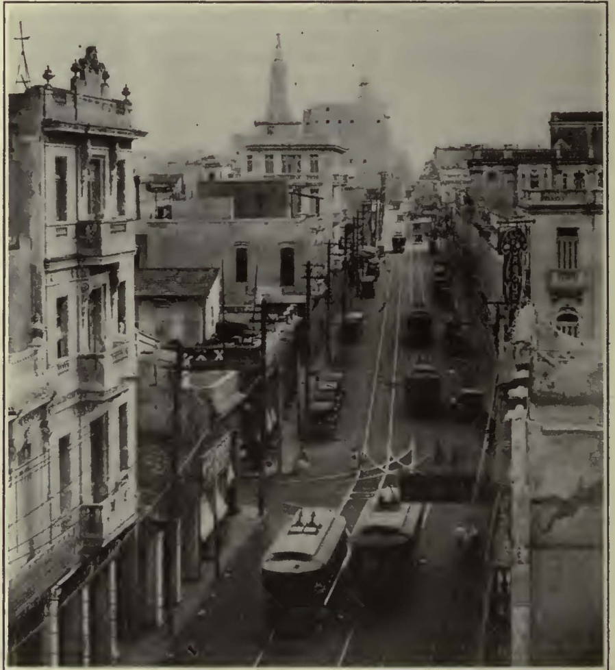
Small Single-Track Cars and a Double Overhead Trolley Wire System Are Characteristic Features of Electric Railway Operation in Havana
