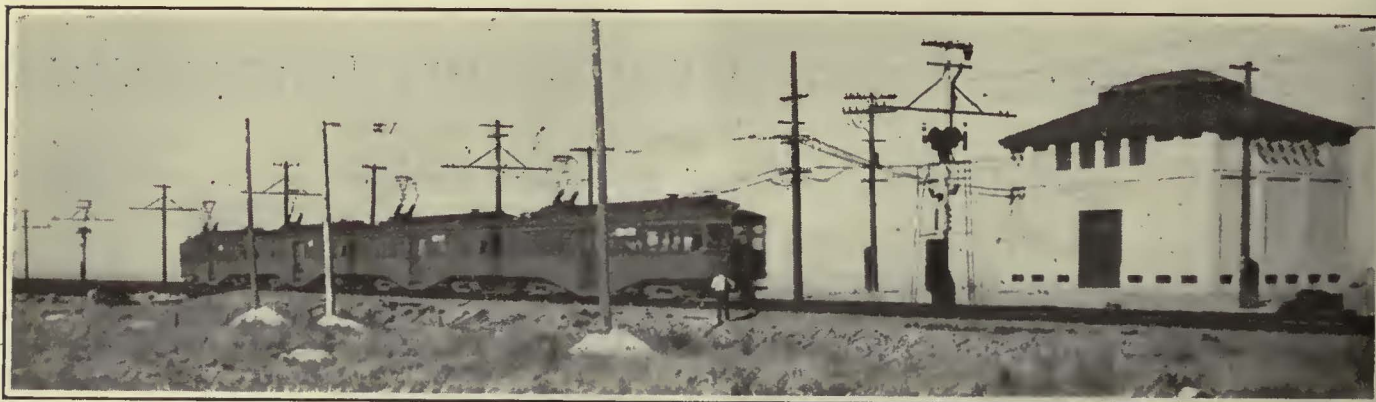
A Four-Car Train of the Key System Transit Company Passing the New Substation Located at the End of the Earth-Filled Portion of the Key System Pier Well Out into the Middle of San Francisco Bay
