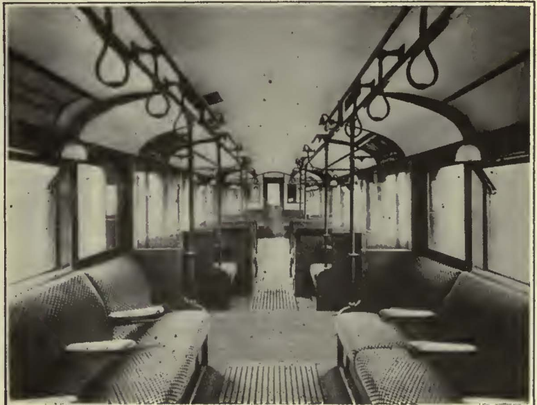
Interior of C. L. R. Cars After Alterations
