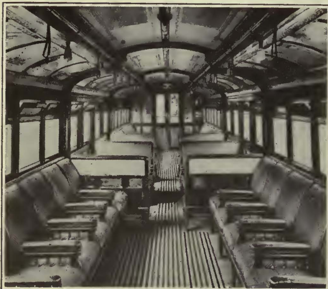
Interior View Before Alterations Had Been Made
