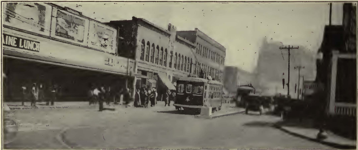
Island Platforms with End Lights, Installed by City, Speed Boarding and Alighting
