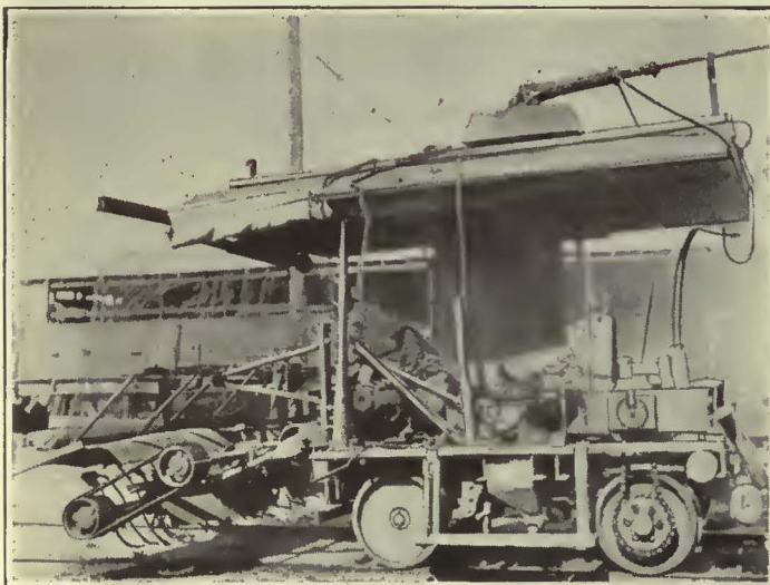
Weed Whipper Used by Texas Electric Railway
