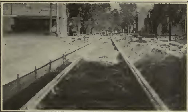
Placing the Gravel and Bringing the Track Up to Grade
