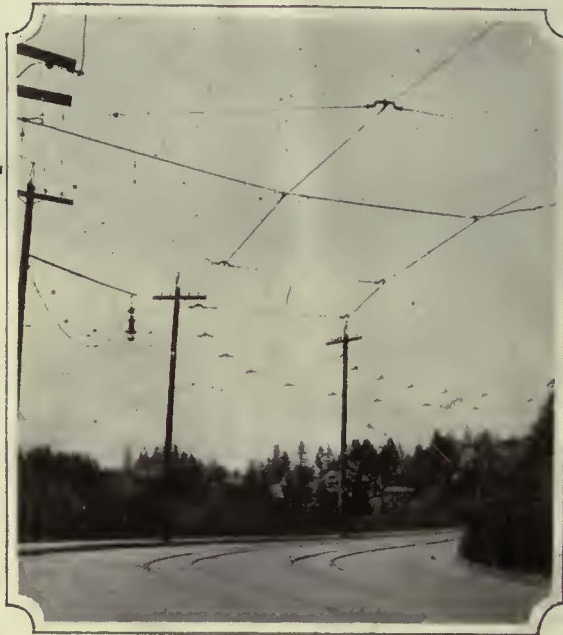
This photograph shows part of the Phono-Electric installation on the Portland Electric Power Company's Council Crest line. Phono's exceptional wear resistance and high tensile strength make it especially valuable on sharp curves such as this.
