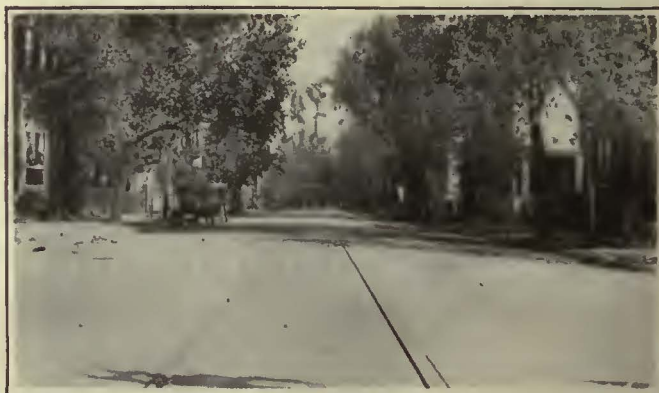
A Cold Asphalt and Crushed Rock Mixture Was Used for the Paving
