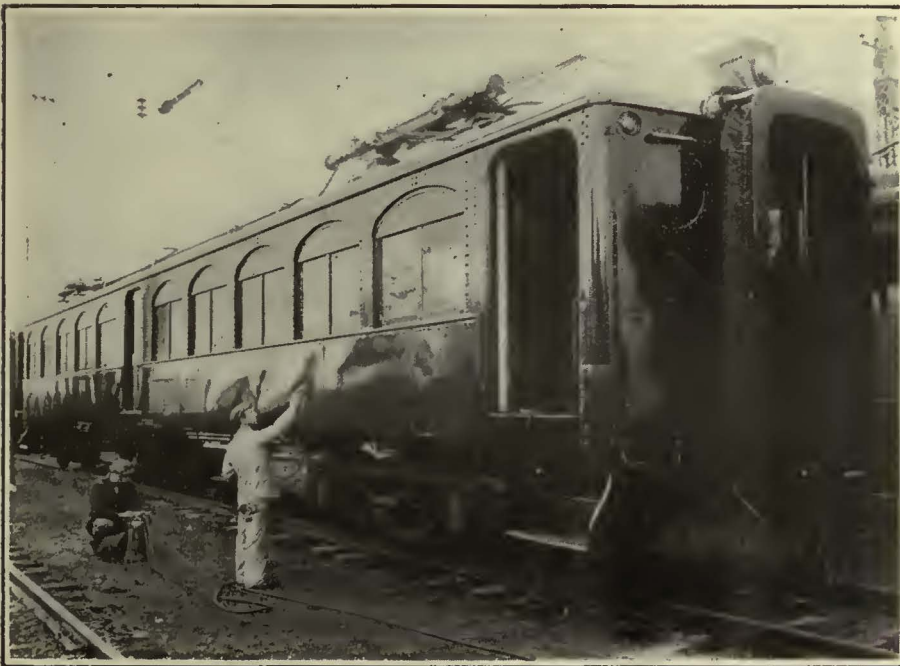
Time for Painting Exteriors of Cars Was Reduced One-Third by the Spray Method
