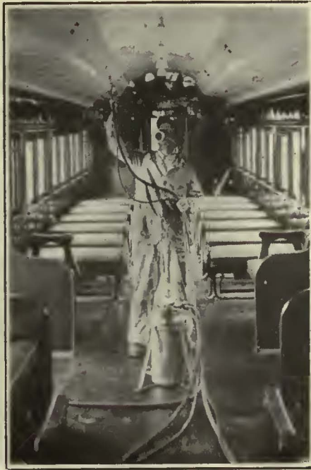
The Operator Uses a Respirator While Spraying the Interior Headlining
