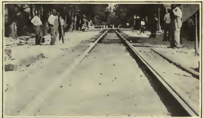
Placing the Gravel and Bringing the Track Up to Grade
