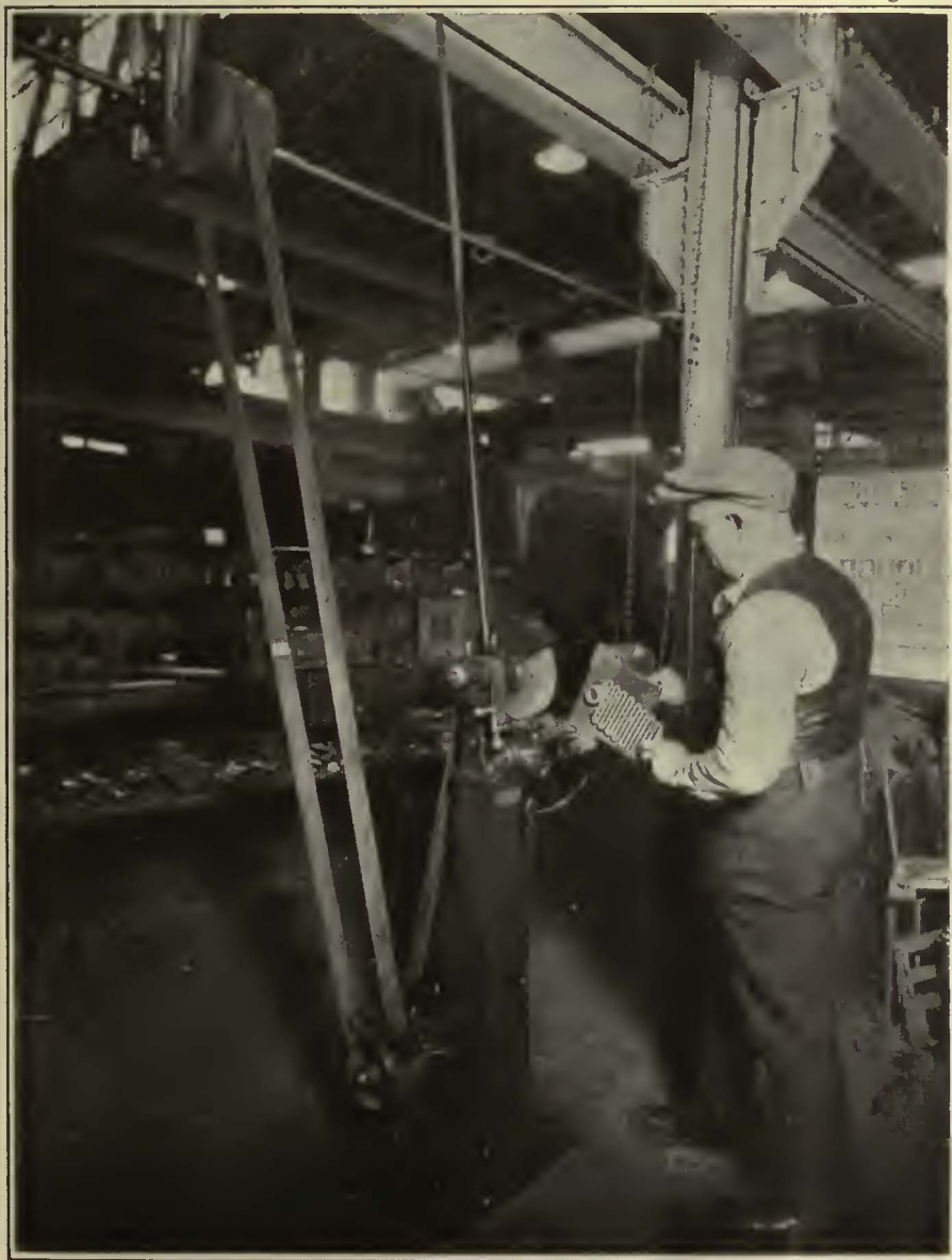
A Special Attachment to a Standard Grinder Is Used When Grinding the Contact Face of a Resistance Grid
