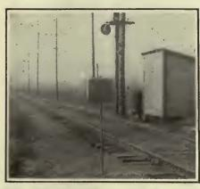
Better Protection for Trackmen Has Been Secured on the Lines of the T. H., I. & E. Traction Company by the Use of Metal Markers Instead of Cloth Flags
