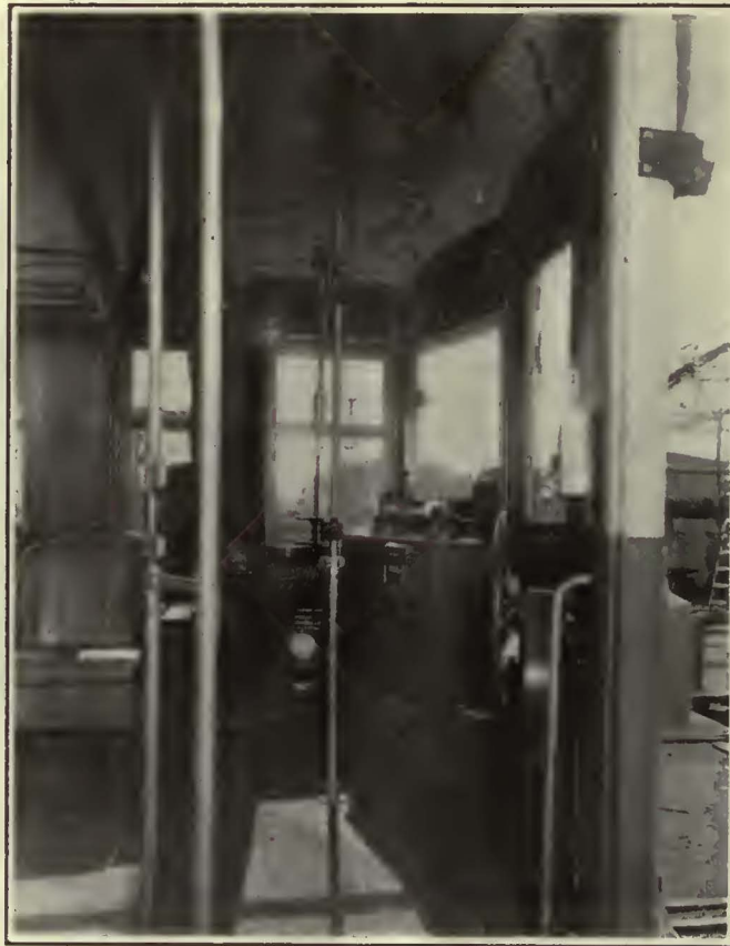
View from the Front Side Door of the Control Equipment on One of the New Cars
