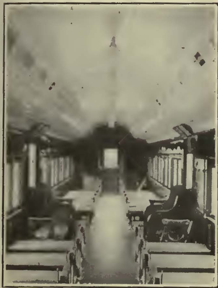
The Worn Aisle Is Filled In with Composition Flooring and Is Then Sprayed Red. New Type of Gas-Filled Lamps Are Installed
