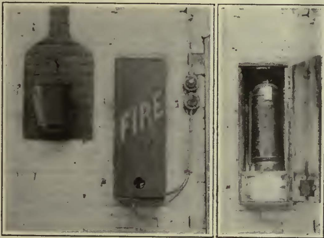
Fire Extinguisher Container Is Here Shown in Both Open and Closed Positions to Indicate Simplicity
