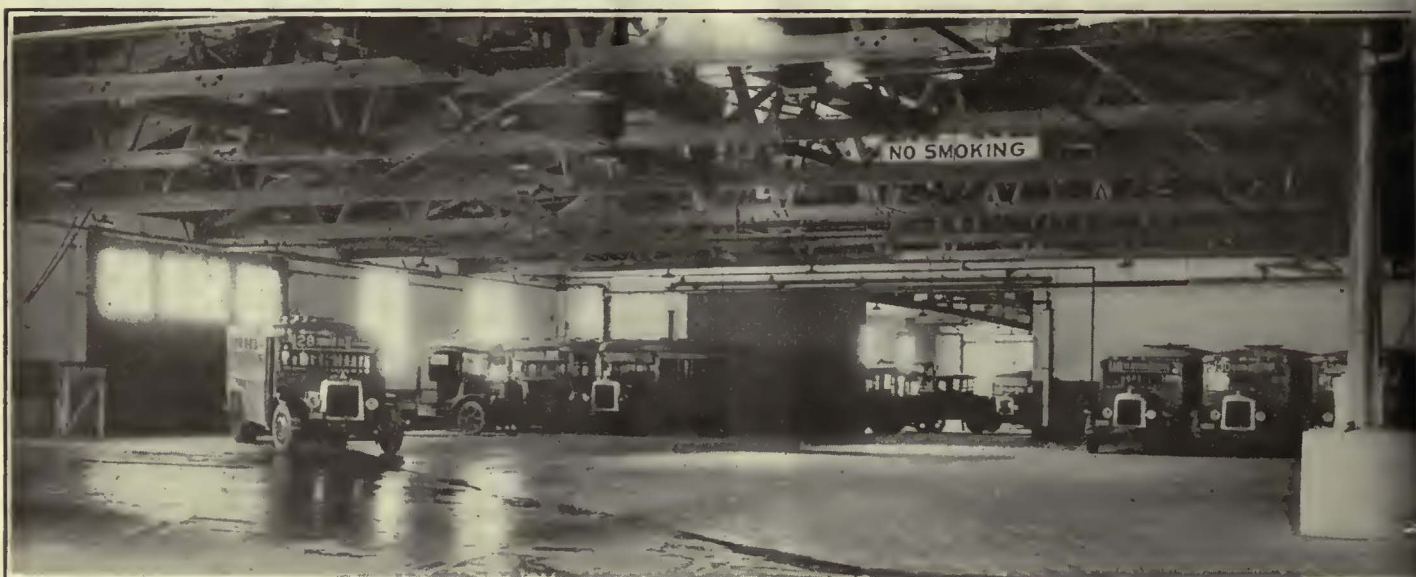
Carefully Designed Roof Trusses Render Interior of Lake Street Garage Remarkably Fr...
