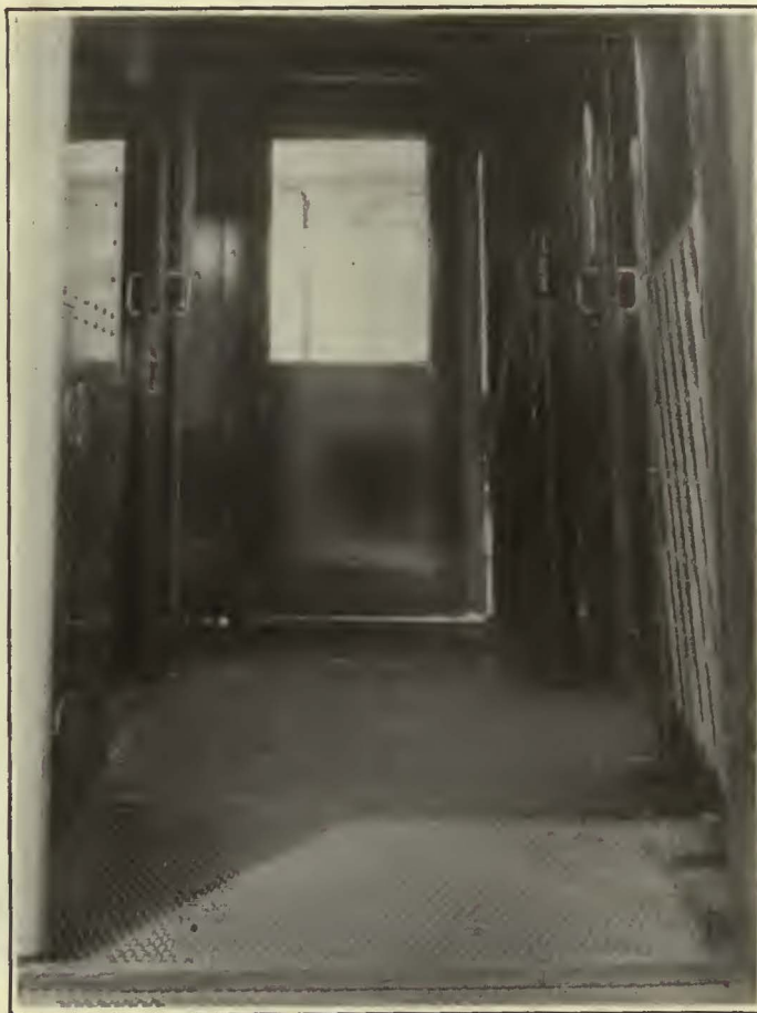
Safety Treads Do Away with the Necessity for Rubber Mats on Platforms. A New Steel Door Has Been Installed
