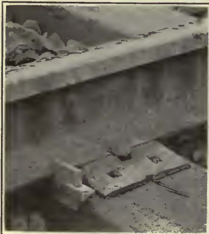
Rail Anchor After Installation
