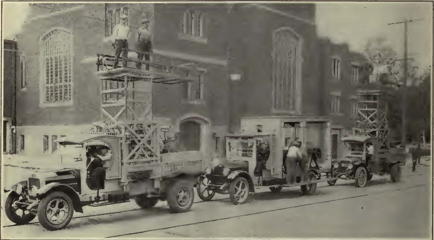
By Use of the New Reel Truck Together With two Tower Trucks, Trolley Wire Can Be Taken Down and New Wire Installed at the Same Time without Interrupting Traffic
