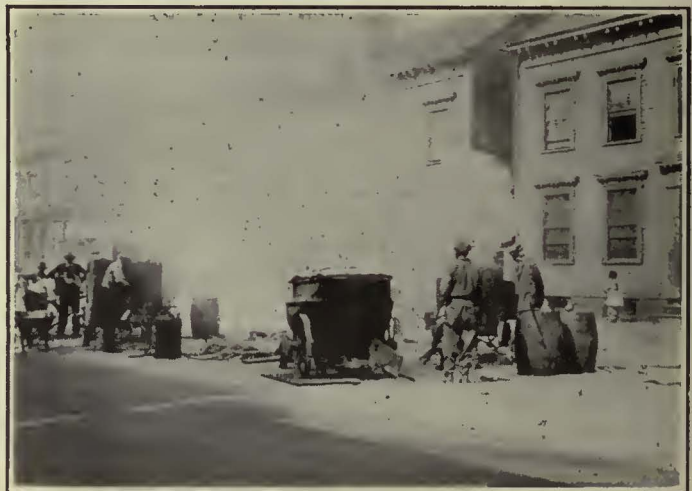
Pouring Hot Mastic Filler between the Granite Paving Block
