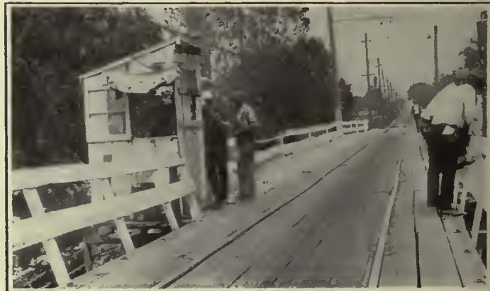
Watchman's Shanty with Long View in Both Directions, from Which Signals Were Controlled
