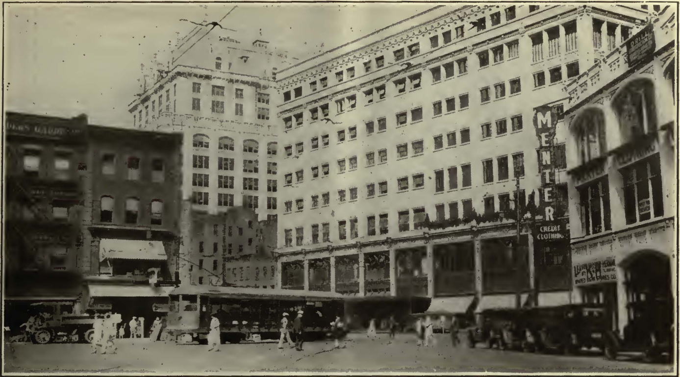
At the Intersection of Washington and Market Streets, Newark, N. J. Buildings on the Southeast and Northwest Corners Were Demolished in Order to Eliminate a Bad Jog, Thereby Making Possible the Installation of a Diagonal Crossing and Permitting Through Railway Operation on Washington Street
