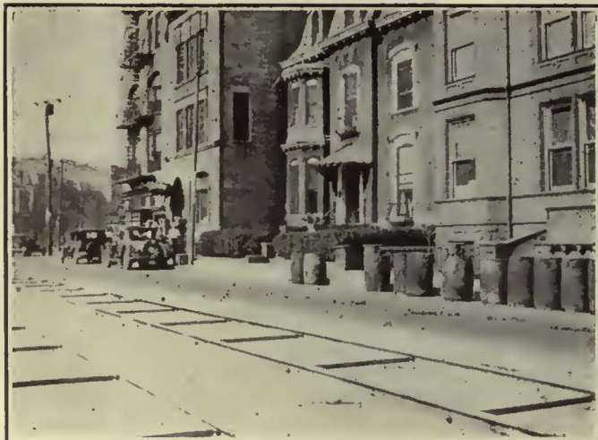
Concrete Was Poured on the Ballast Even with the Tops of the Ties
