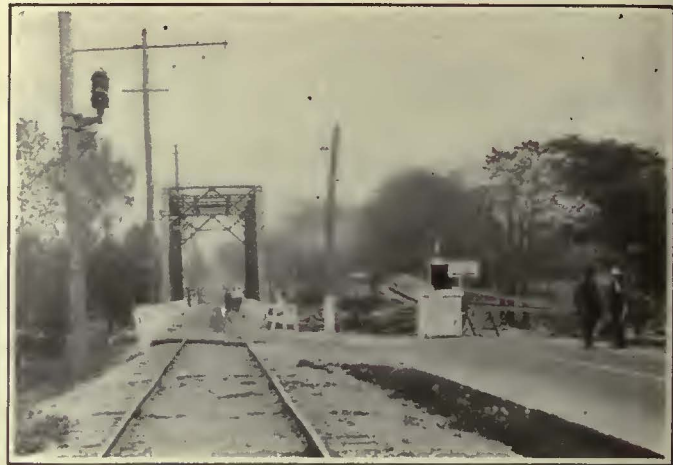
Railway and Highway Signals Interlocked Near Richmond, Ind., While Vehicular Traffic Temporarily Used the Bridge of the T. H., I. & E. Lines
