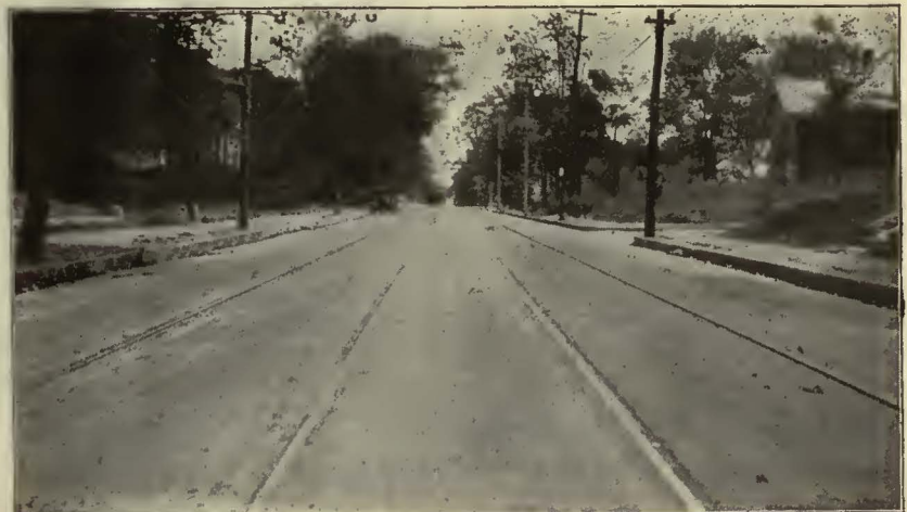
A section of the track of the Nashville Railway & Light Co., Nashville, Tenn. This track is cushioned with Carey Elastite Rail Filler.
