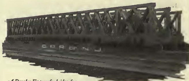
A Douglas Fir transfer bridge for car floats of the Central Railroad of New Jersey.
