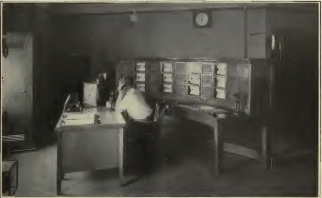
The Heart of the Supervisory Control System
