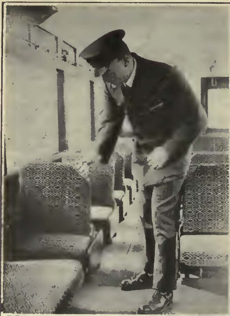
At Left, Spring-Cushion, Plush-Upholstered Seats Are Being Installed on Cars of the London County Council Tramways to Encourage Traffic. At Right, Installation of Additional Lamps Gives 60 Per Cent Better Illumination Inside the Car
