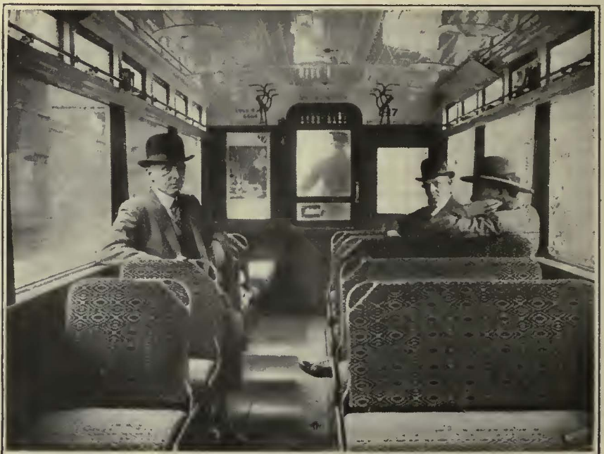
At Left, Spring-Cushion, Plush-Upholstered Seats Are Being Installed on Cars of the London County Council Tramways to Encourage Traffic. At Right, Installation of Additional Lamps Gives 60 Per Cent Better Illumination Inside the Car
