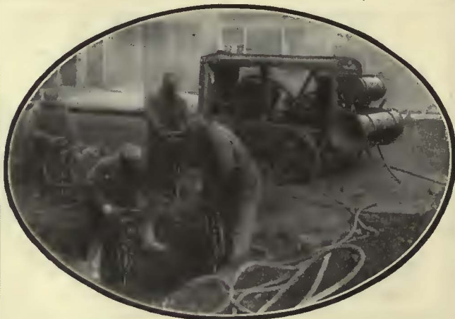
Sullivan Busters and Sullivan Portable Compressor breaking concrete in Philadelphia. Mazzola-Marano, who were contractors on this job, ran 4 "DW-221" Heavy Busters at a time with the "WK-314."
