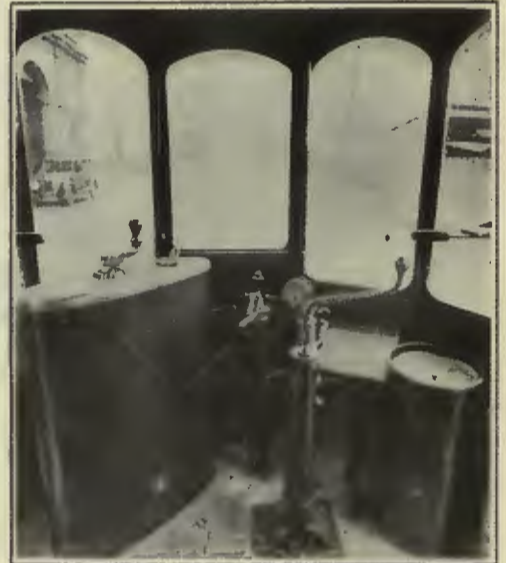
Many Features Characteristic of American Electric Railway Practice Are Embodied in the Design of This New Single-Deck Car of the Glasgow Corporation Tramways. At Right, Arrangement of Equipment on the Platform Follows the Usual American Practice
