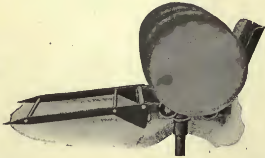
This Type of Skid and Barrel Drainer Is of Great Assistance for Emptying Contents of Barrels
