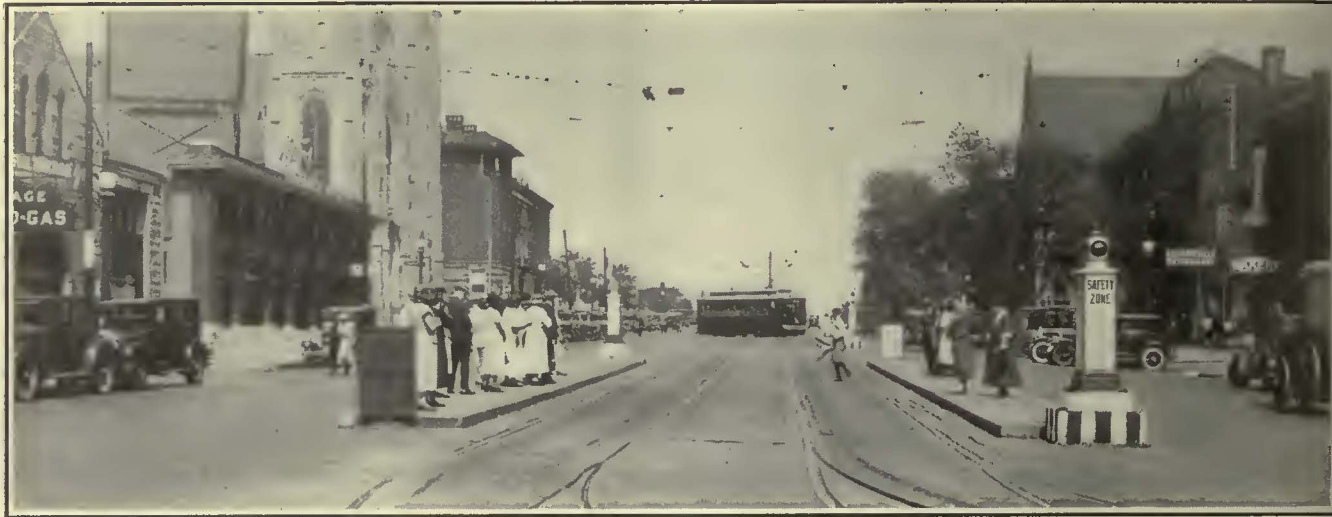
Some of the Streets in Baltimore Are Equipped with Raised Platforms. The Entering End of the Platform Is Protected with a Safety-Zone Light Post, with Conspicuously Marked Base, and the Leaving End with a Substantial Frame Containing a Safety Poster. This View Is on North Charles Street
