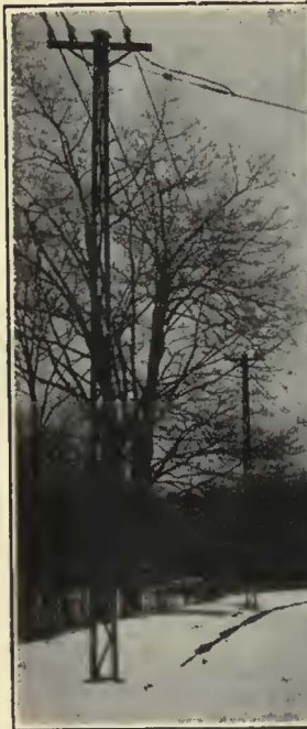
Installation of the Grand Rapids Street Railway Co.
