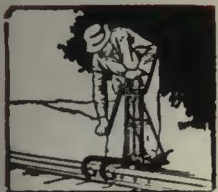
Track and Bonding Drill
