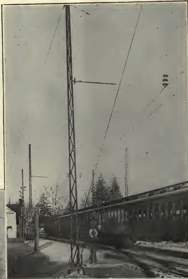
Installation of the New York, New Haven and Hartford Railroad Co.
