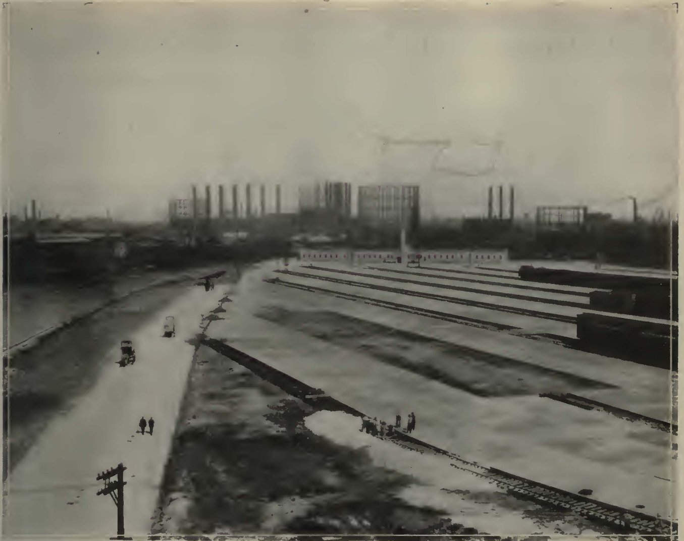
The spacious team yard of the Atchison, Topeka and Santa Fe Railway, Chicago, completed 1926. Paved with concrete 10 inches thick.
