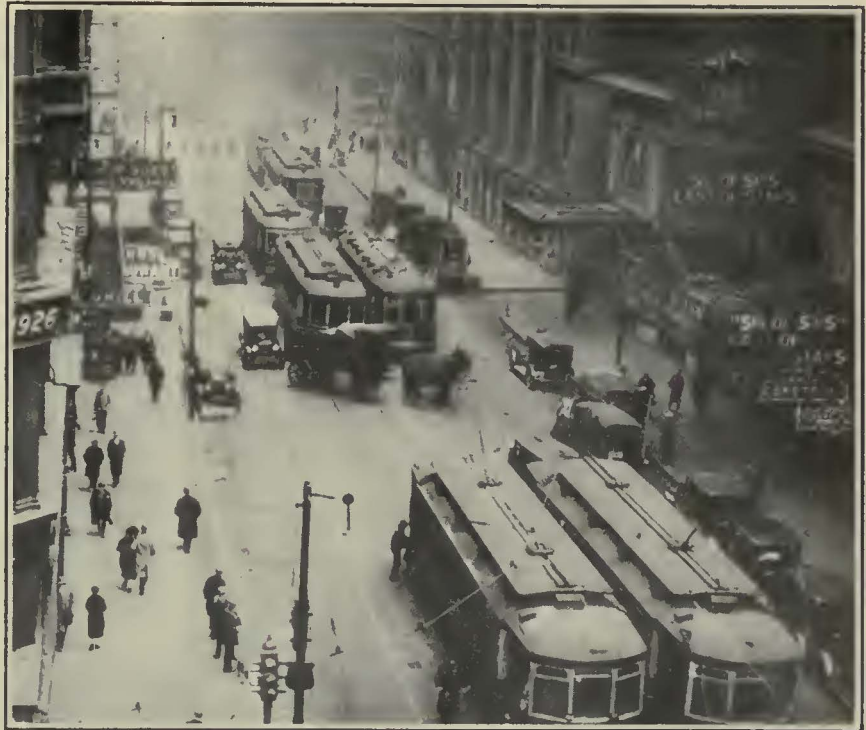
With the Abolition of Left Turns in the Chicago Loop, Midstreet Turns Are Permitted, but with Inevitable Delays, as Illustrated
