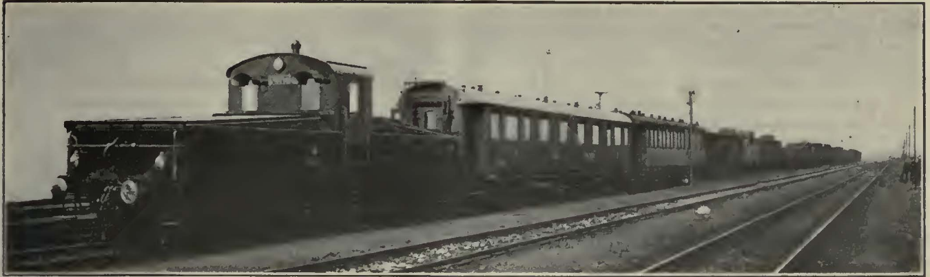
Storage Battery Locomotive Hauling Train at Wilson Terminal, Prague
