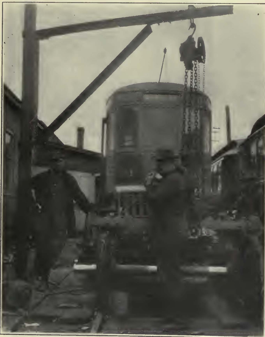
Truck Frame Suspended on Outdoor Derrick Chain Hoist
