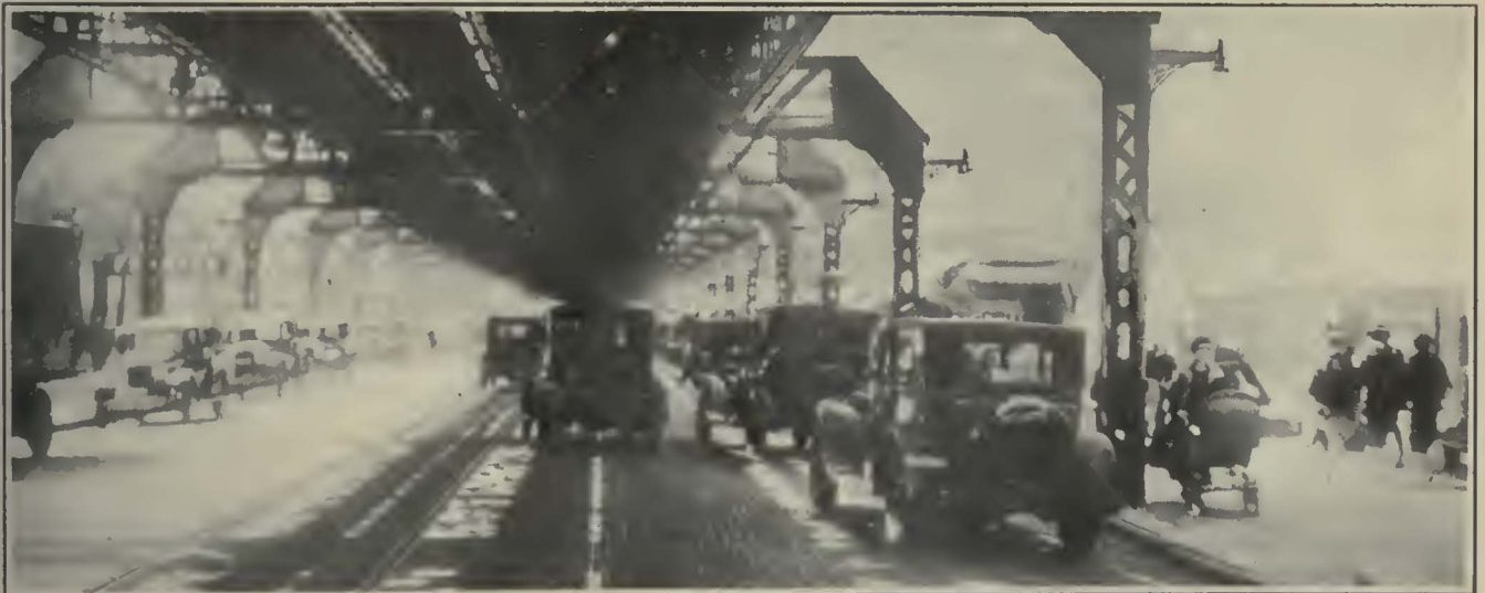
Curb Supports of the Elevated Structure on 63d Street, Chicago, Are an Important Improvement Which Benefits Street Traffic
