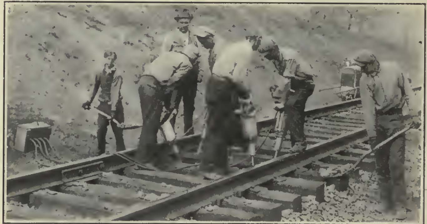
The Power Plant of the Syntron Electric Tie Tamper Weighs so Little that It Can Be Carried by Hand from Place to Place. A Battery of Four Electric Tampers at Work
