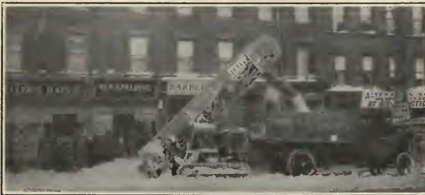
Above, Snow Loader Removing Snow Which Has Been Swept and Plowed to the Side of Car Tracks. At Right, Heavy Type Snow Loader
