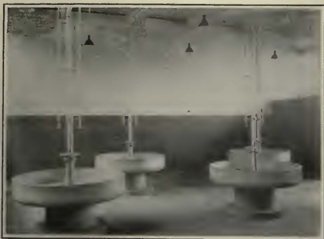
Circular Wash Fountains Are Provided for Workmen
