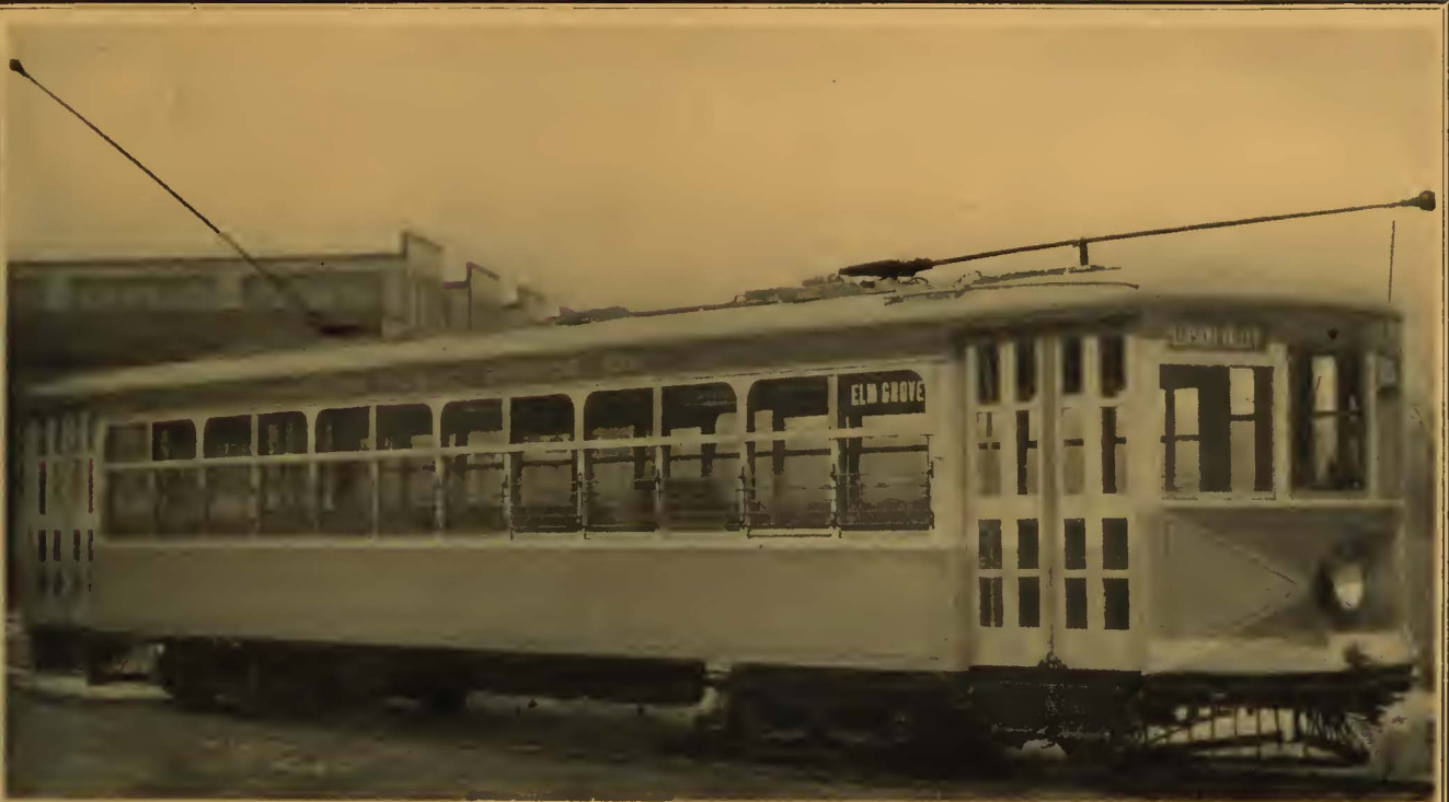
15 light-weight, one-man, two-man cars built by Kuhlman. Mounted on Brill 177-E trucks.
