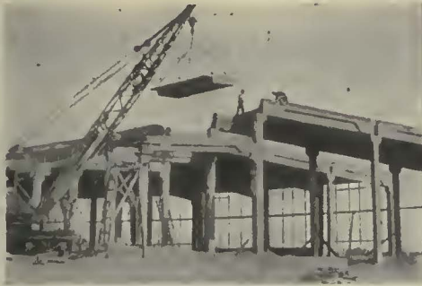
Lowering roof slab unit, Round House, Stockton, Calif.
