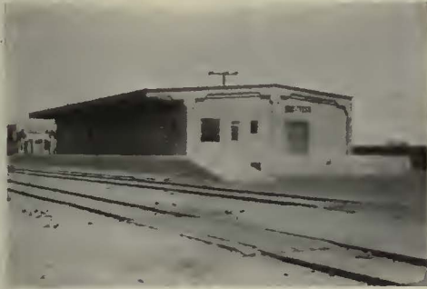
Oil House, all precast concrete units, except platform, Sacramento, Calif.
