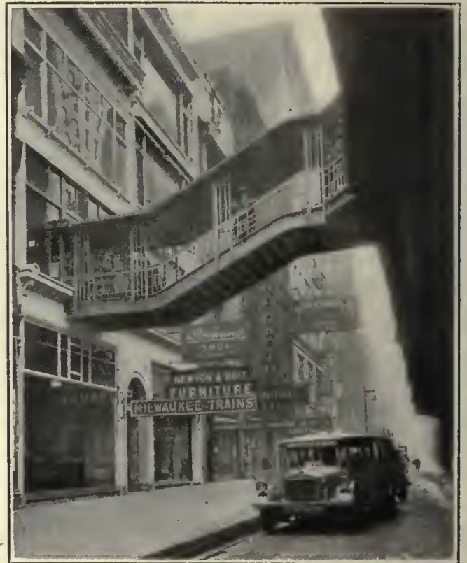
New North Shore Station on Wabash Avenue in Chicago Connects Directly with the Adams and Wabash "L" Station
