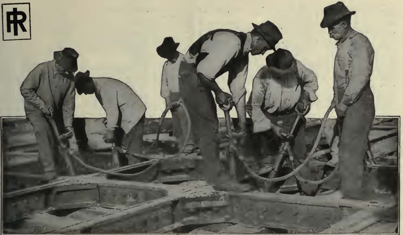
4 Pneumatic Tie Tampers at Work on a Crossover
