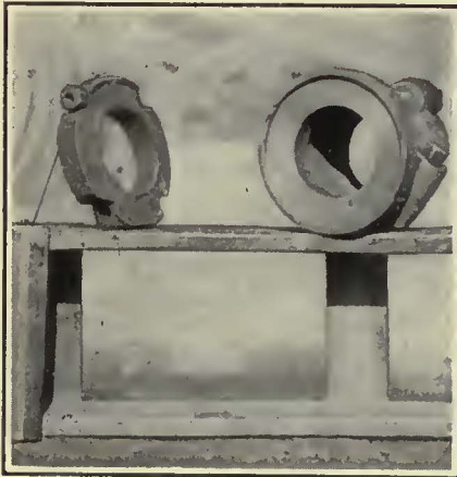
Old Collar on Left and New Adjustable Dust-Deflecting Collar on Right
