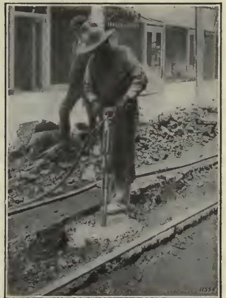
Breaking out heavy concrete base with "I-R" CC Paving Breaker
