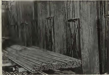
Trolley Pole Stock In Nuttall Store Room
