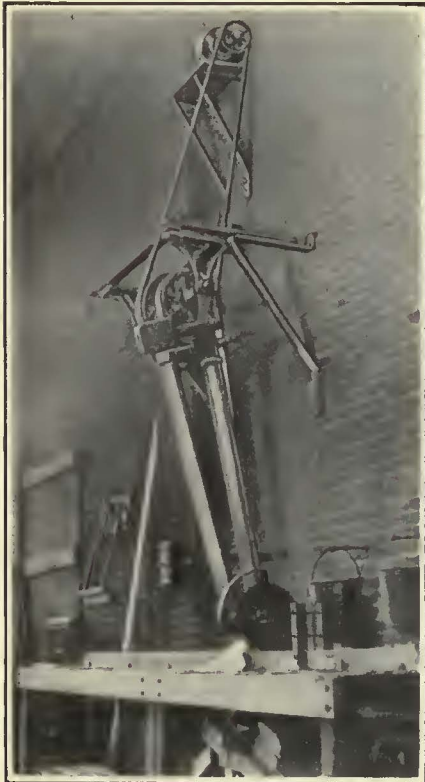
Circular Swing Saw Belt Driven by an Air Compressor
