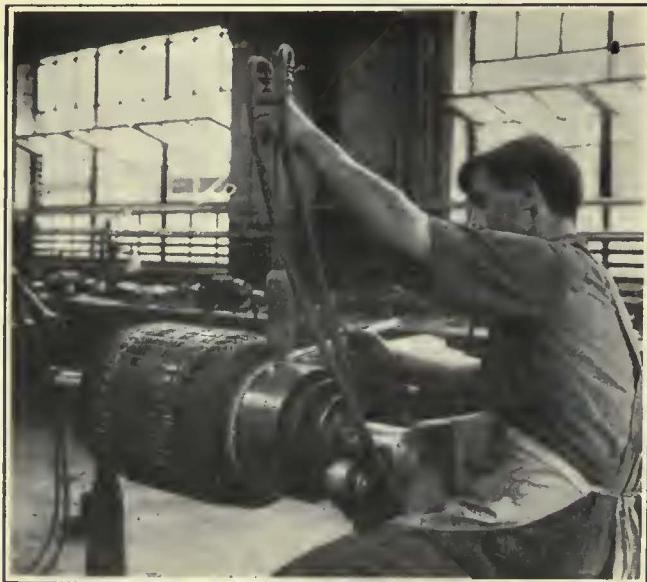
Solderlug an Armature at the Top with a Self-Heated Iron
