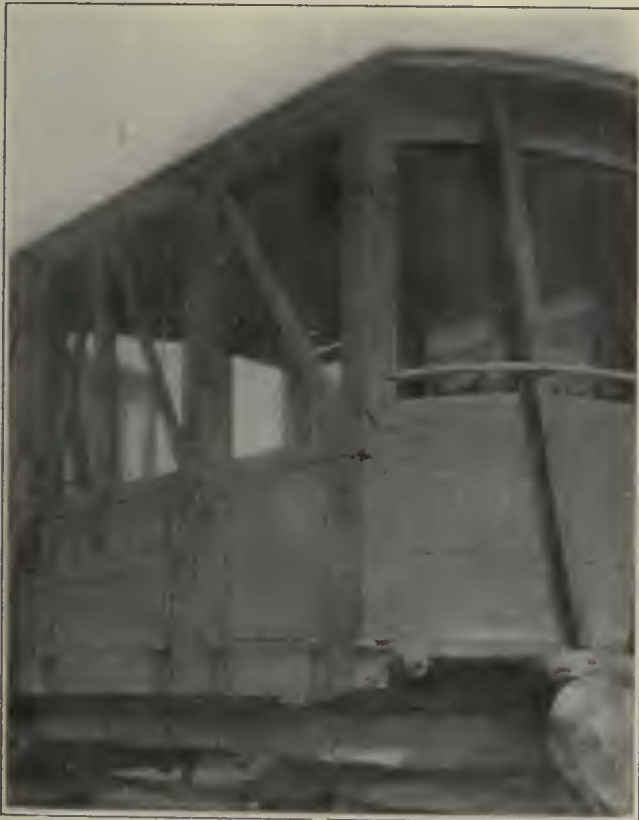
Refuse Car Has Hinged Section of Solid and Screened Parts
