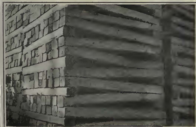
Method of Piling Timber for Storage at South Boston Creosoting Plant. Untreated Ties Are Shown at Left and Treated Ties at Right
