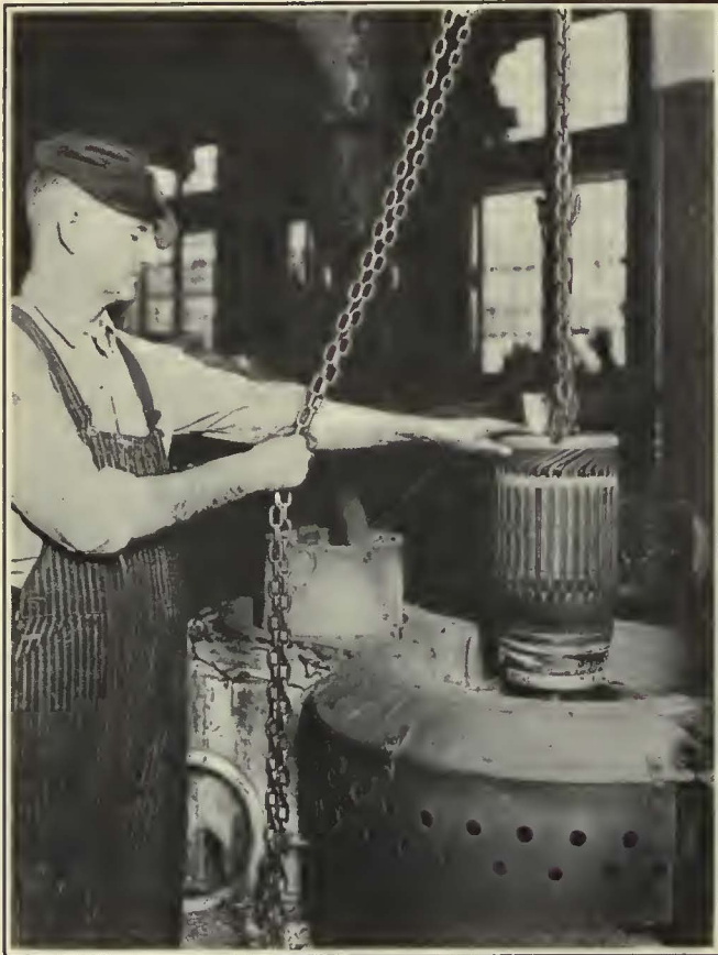
Dipping Armature to Solder Leads
