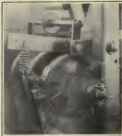
Close-Up View of the Brake, Which Is of the Automobile External Contracting Type. It Is Held Closed by Weights on the Lever, but Is Operated as the Tension on the Wire Turns on the Pulley Shown Just Above the Brake
