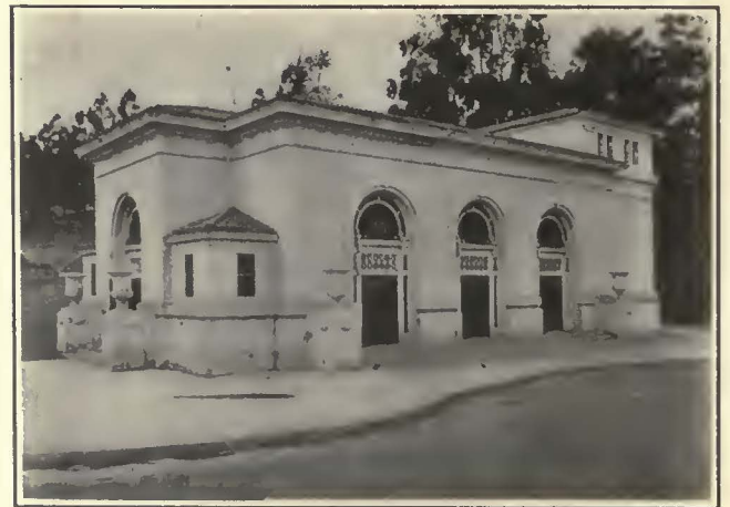
Type of Station Used at Intermediate Points of Tunnel. Elevators Lower the Passengers to the Train Level
