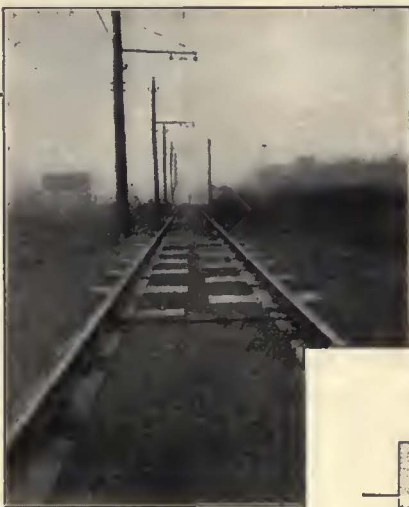
View on the main line of the P. H. B. & N. C. Railway, at Ziegler Station, Pennsylvania, showing the interesting stages from the wooden cross-tie to the finished track insulation system. Note first the square concrete blocks, then the tie extended toward the center of the track, and finally the cruciform ties, shown in staggered rows in the perfected system.
