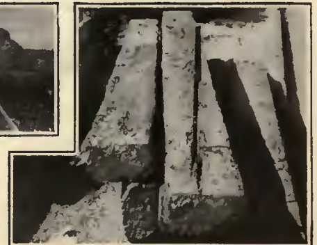
Creosoted Ties Installed in 1895 on the Property of the Georgia Railway & Power Company Were Removed in 1926. A Large Majority Were Found to Be in Good Condition After 31 Years Service
