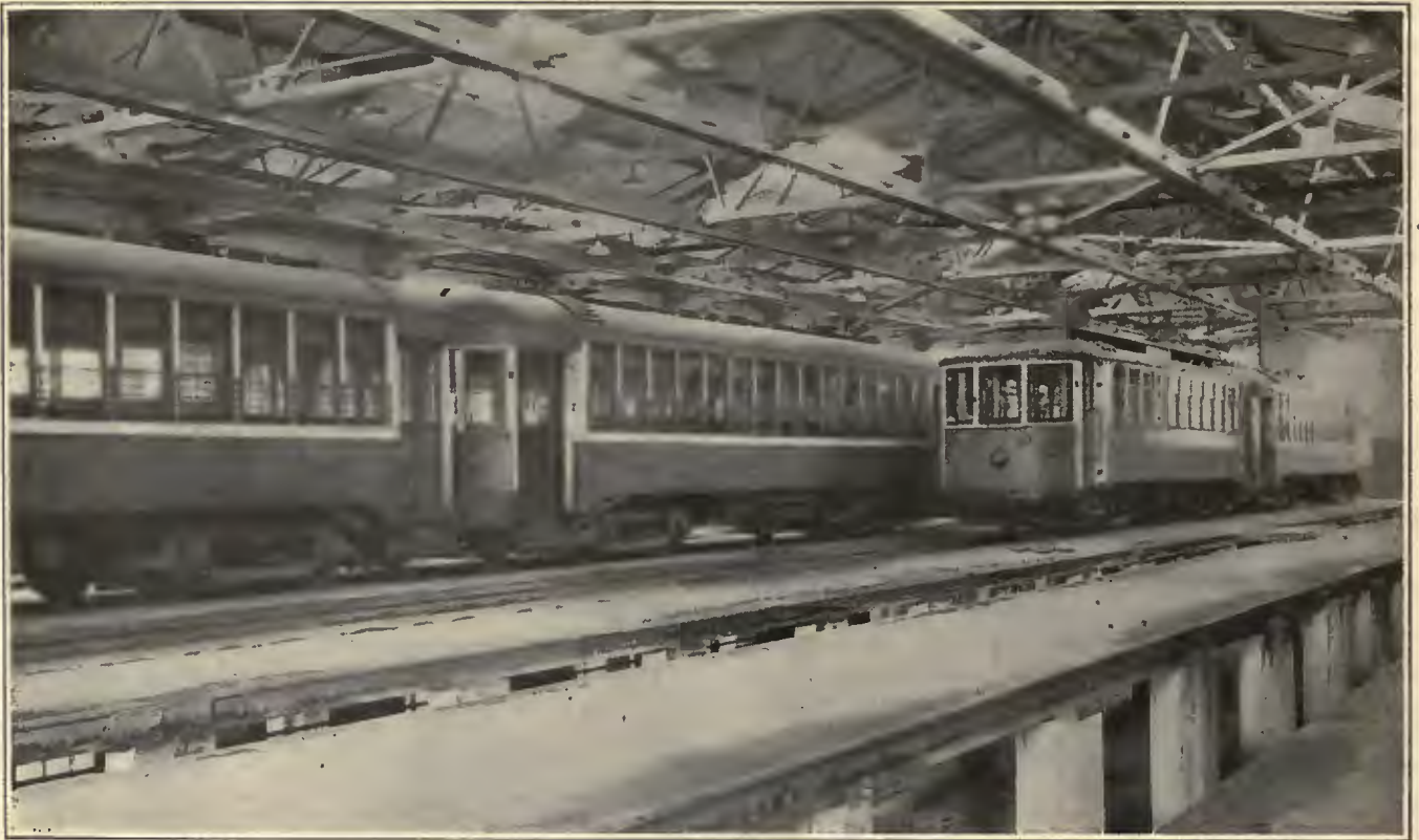
In the Operating Carhouse the General Floor Level Is 4 Ft. 6 In. Below Ground, with the Rails Supported on Reinforced Concrete Columns. The Space Between the Two Rails of Each Track Is Left Open to Facilitate Inspection of Running Gear of Cars
