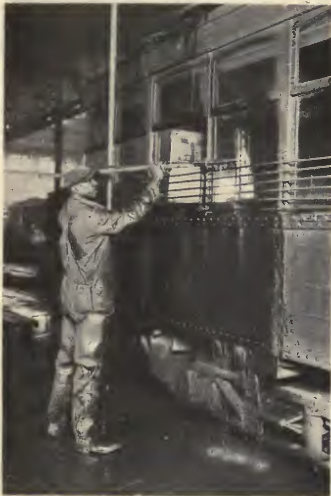
Method of Using Strip Brush to Clean Window Glass Behind Guard Rails When Rotating Brushes Do Not Remove Mud
