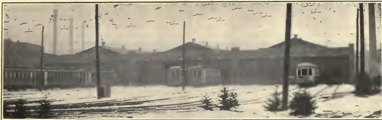
Three Bays of Five Tracks Each Accommodate a Total of 55 Cars Under Cover in the New Operating Carhouse at Waterbury
