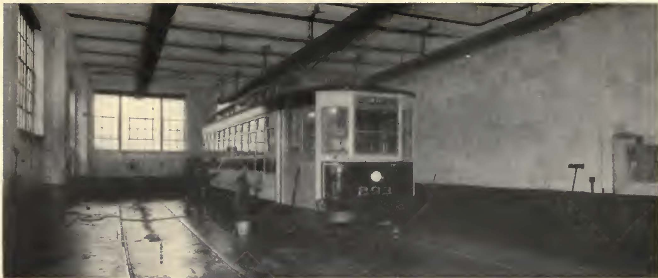
General view of the wash room at the West Farms carhouse of the Third Avenue System
