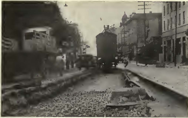
Preparing new track foundations in West Liberty near Pioneer Street
