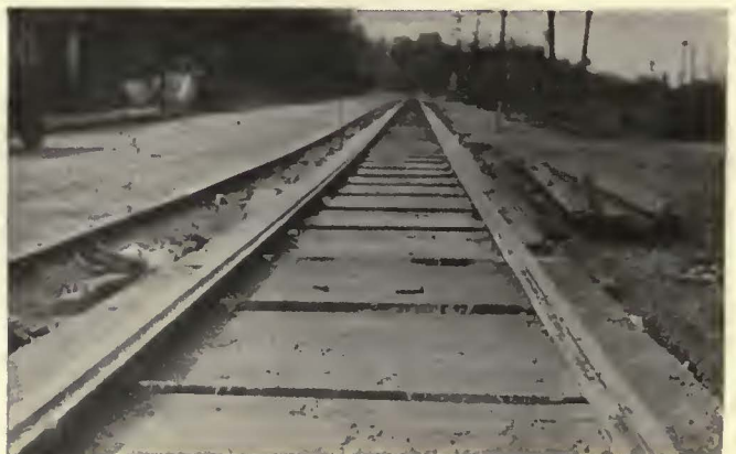
Ballast in place on section of track on McClure Avenue
