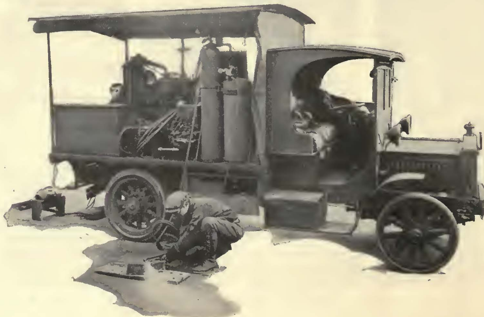
Cutting with the oxyacetylene torch produces savings in track maintenance
