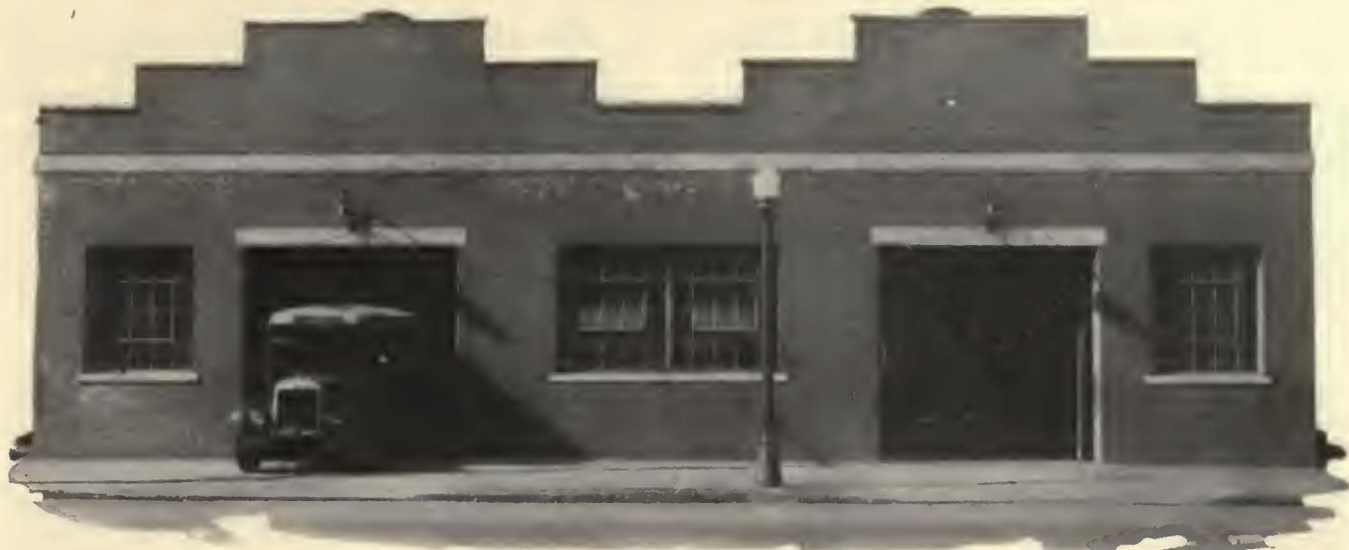
Just to the north of the main carhouse and repair shop in Chattanooga is a 70x200-ft. garage recently built by the Tennessee Electric Power Company
