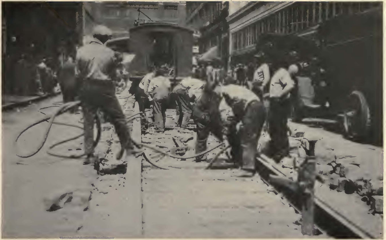
Many small tools such as concrete breakers and tampers are used in track maintenance by the Pittsburgh Railways
