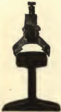
Bar in place on "T" Rail showing Saw Blade Contact
