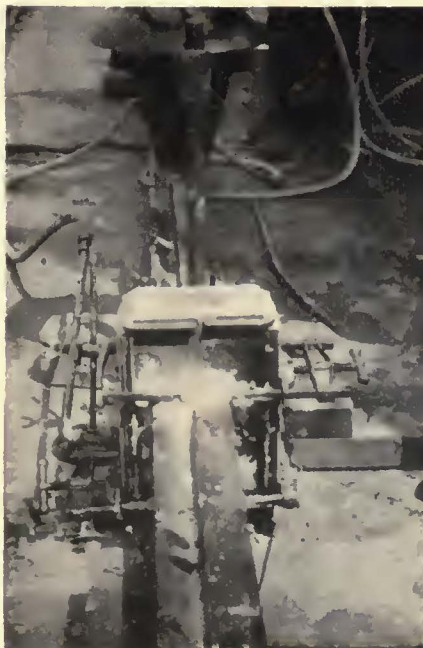
Several rail lengths are thermit welded at the side of the track and then are installed as one piece
