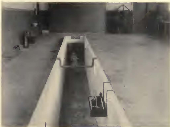
A repair shop feature is a 40-ft. pit with openings along the side for electric lights. The rolling steel door leads into the main storage space
