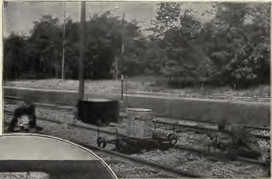
Brazed Bonding with Type SR Outfit
