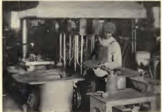
Relining an armature bearing in the new babbitt department of the Pittsburgh Railways
