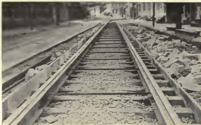
Concrete used in track construction on East Street
