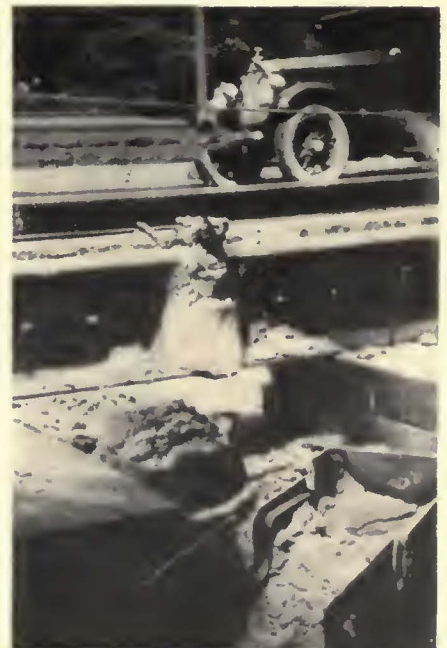
Several rail lengths are thermit welded at the side of the track and then are installed as one piece
