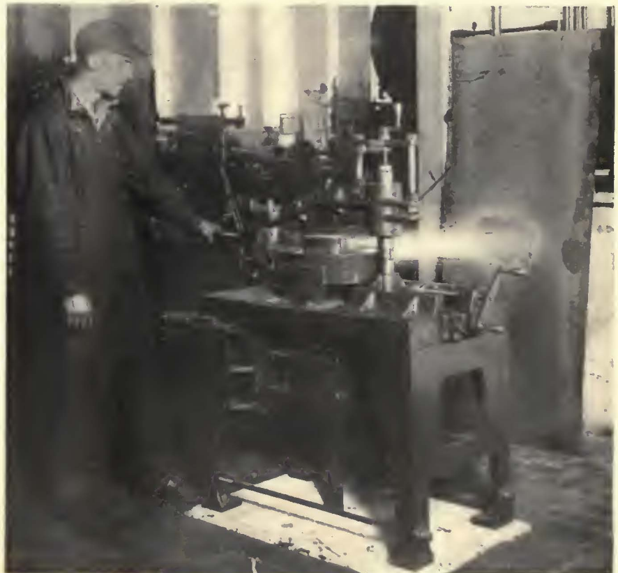
Grinding a shoe head by means of the new machine
