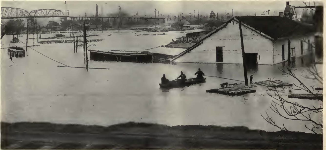
This shows the condition of the company's storeroom at the height of the flood. The men in the rowboat are salvaging poles and materials. At the extreme left a crane is attempting to raise a marooned street car
