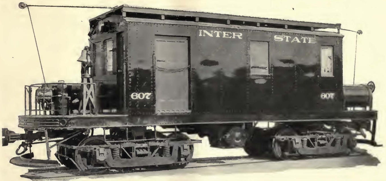
A 40-ton locomotive built by the Interstate Public Service Company from discarded material of two old bridges
