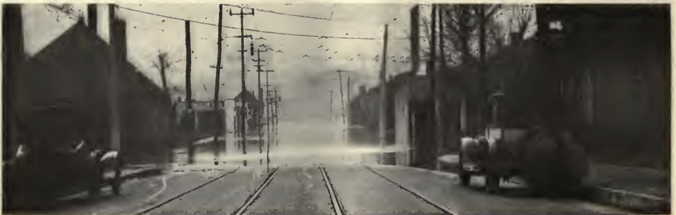
Another deep point was on the Shelby Street car line, where the water covered the tracks about 8 ft.
