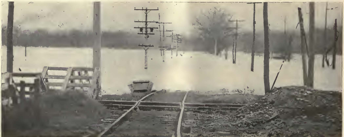
The deepest water was on the Greenwood extension. A stop sign on the span wire may be seen in the distance just above the surface, indicating a depth of about 15 ft.
