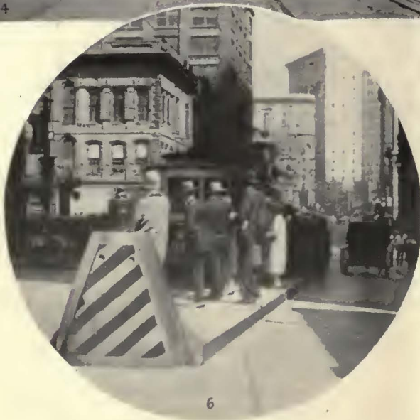
No. 1. Short vertical pieces of rail protect passengers on Cincinnati platforms.
