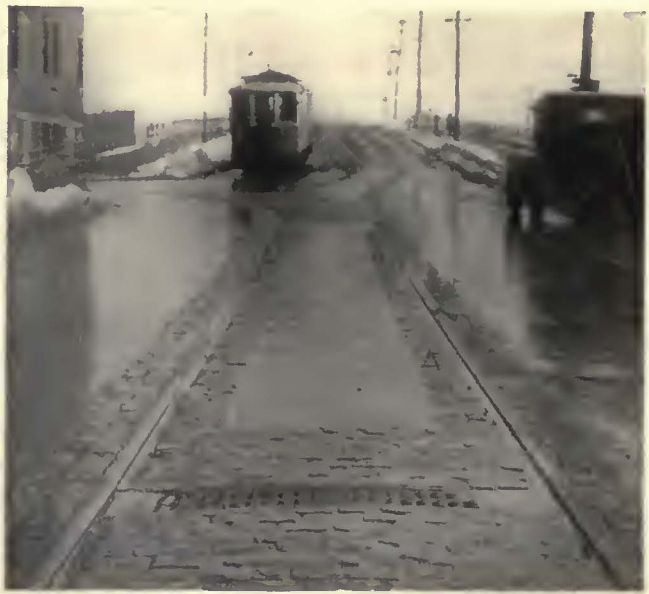
Granite blocks are used for pavement 3 ft. each side of track drains regardless of how remainder of street is paved
