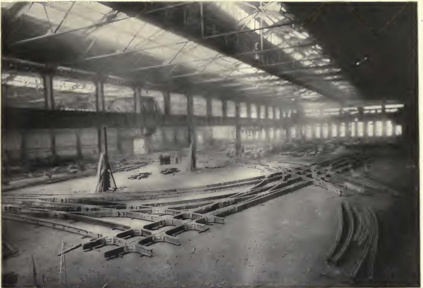
Interior View of One of Bethlehem Track Layout Buildings
