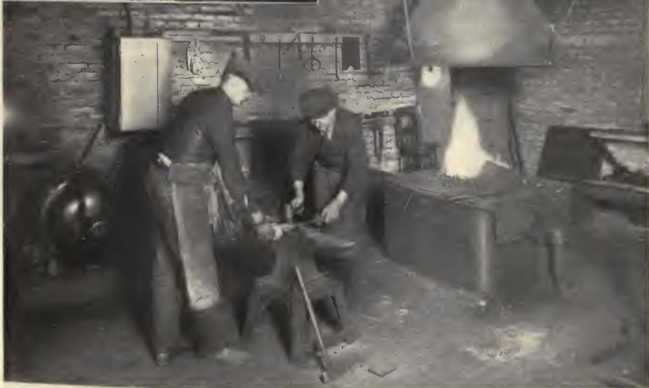
Above—Shop operated by the electrical department to build small special items Below—Special brackets used for mounting are made in the blacksmith shop
