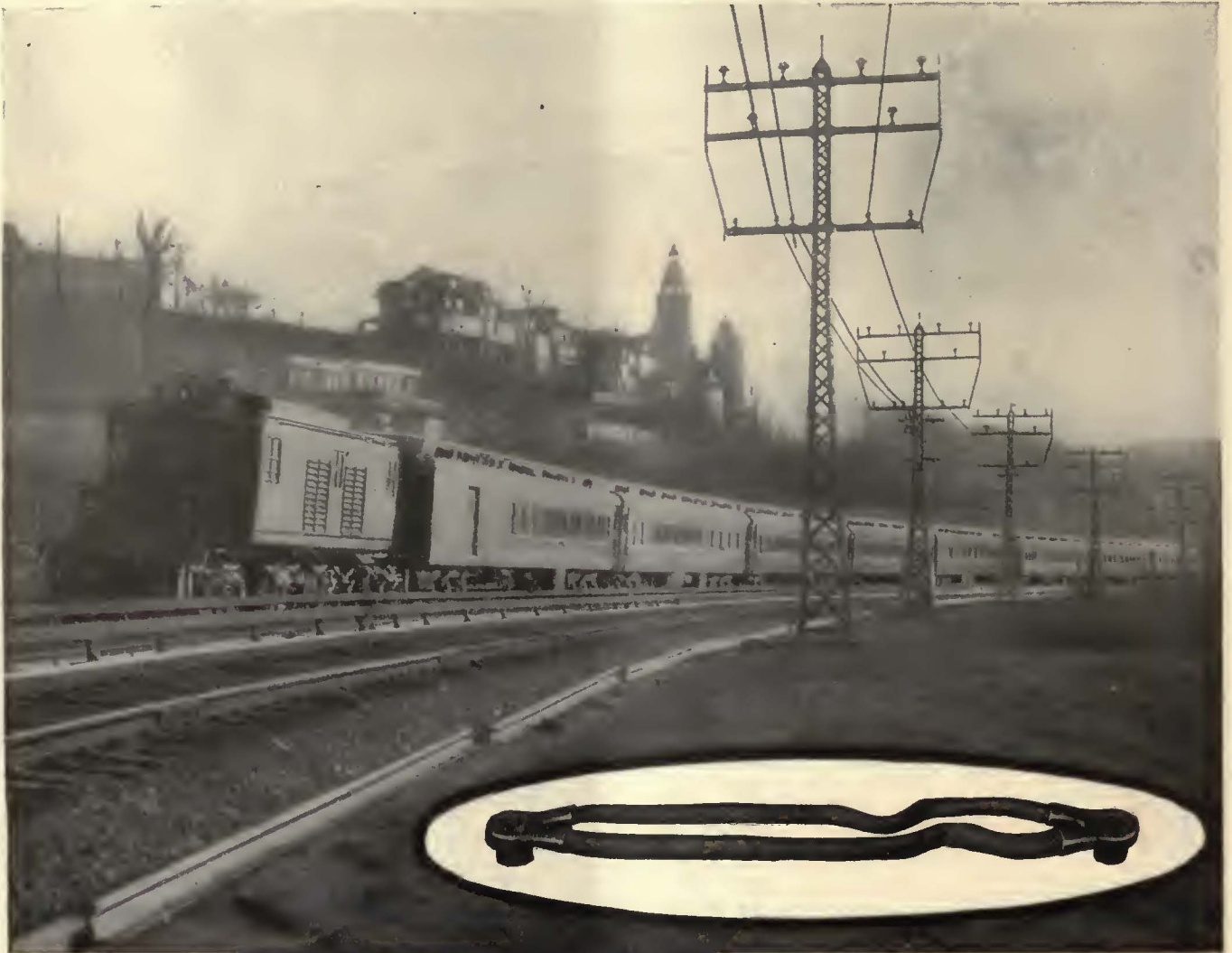
View of 20th Century rounding bend at Marblehead. The New York Central is always among the leaders in modern equipment. Insert shows our type CPO1 Bond used on all main line tracks
