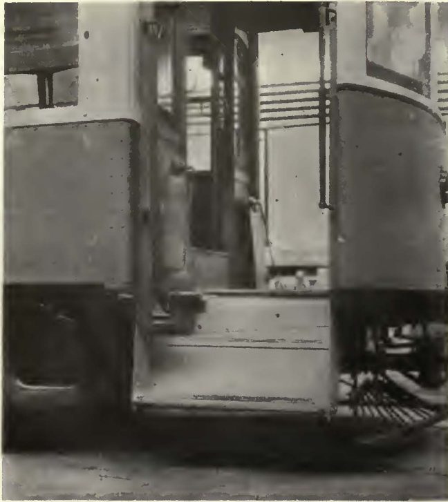
Installation of drop steps in place of fixed wood steps has reduced accidents by eliminating projection and has made passenger ingress and egress easier
