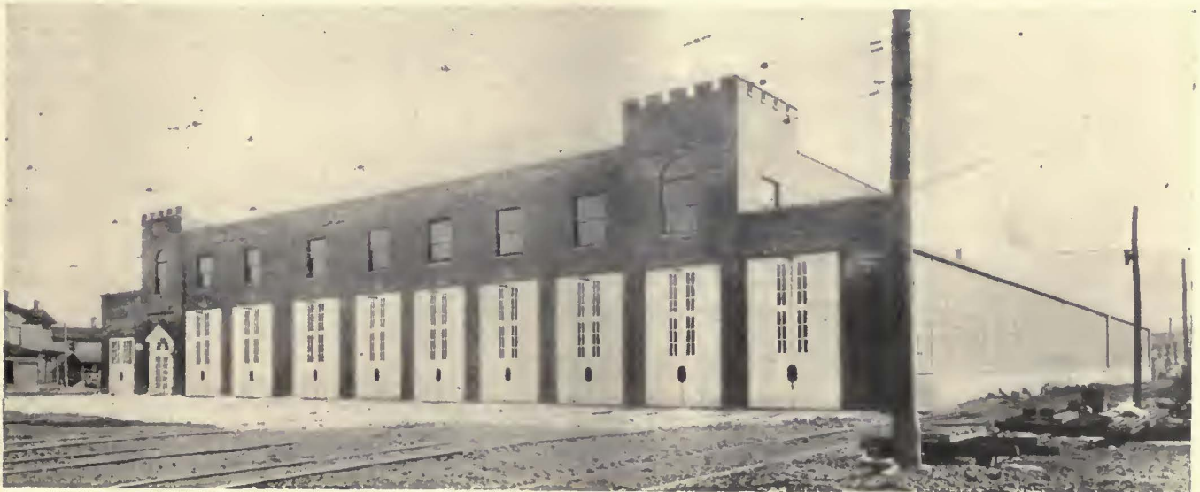
Modern carhouse, shop and office recently completed in Williamsport, Pa. Considerable attention and expense were devoted to architectural design
