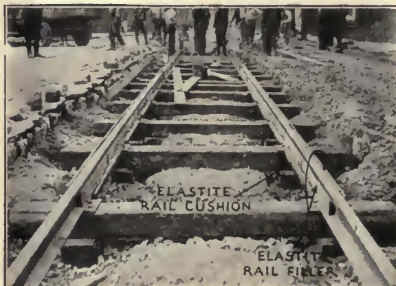
View of the Georgia Power Company Street Railway, on Hunter Street, Atlanta, Georgia. Note the interesting construction features, and the Carey Elastite System of Track Insulation in place.
