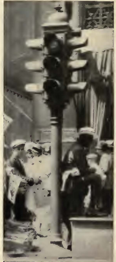
Typical signal light standard in Chicago Loop as it now appears changed to shine in four directions
