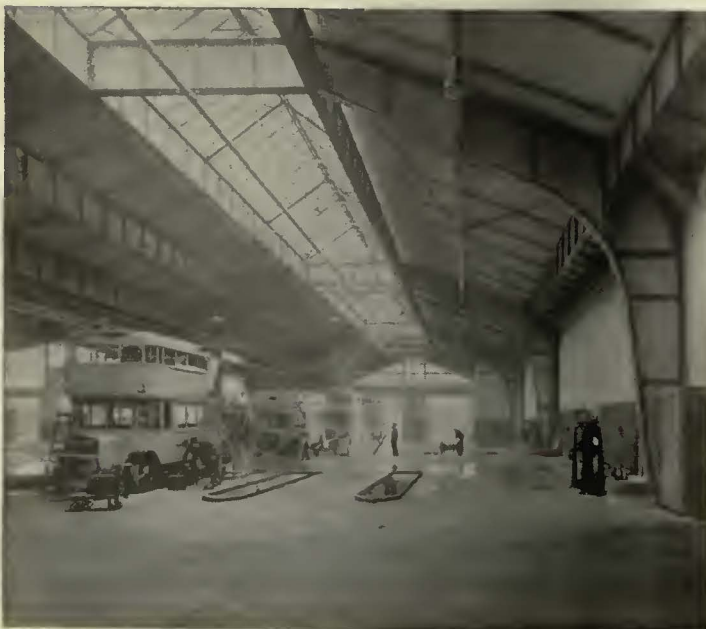
At left, the washing and inspection as seen from the repair pits. At right, column for roof with hot air heater and telephone booth and base protected by wooden curb against sideswiping of bus
