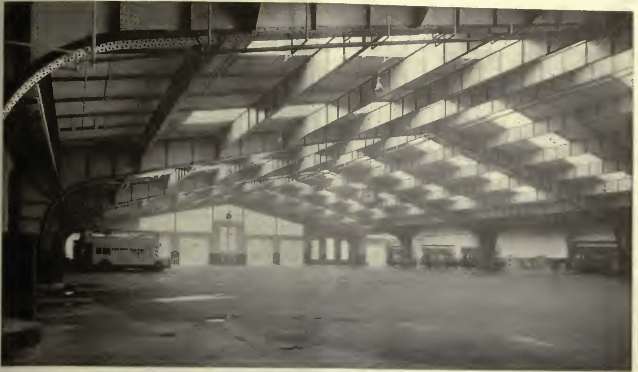
This recent garage at Berlin will hold 200 buses. Washing and inspection are carried on in the bay shown at the right
