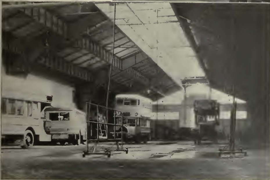
The spraying racks are mounted on wheels so they are adjustable in position. They are connected to the water supply above by flexible hose
