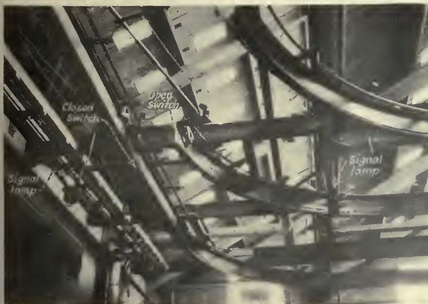
Simple signal system on telfer tracks in Interborough shops prevents derailments
