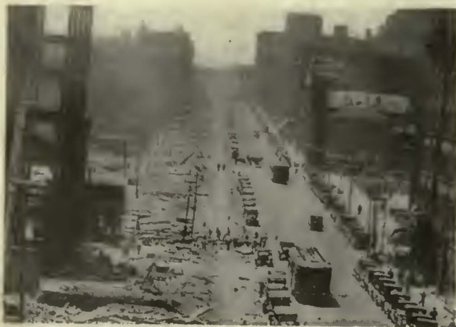
Widening of Olive Street, St. Louis, necessitated the relocation of 3.35 miles of double track of the United Railway
